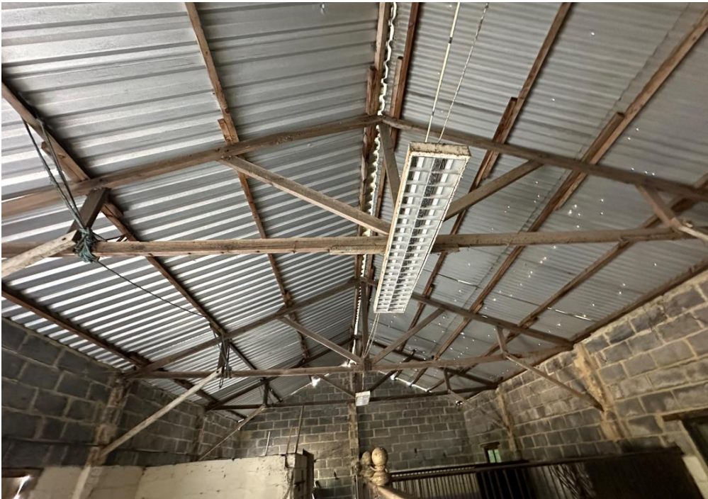
Figure 5; Photographs of showing the timber truss roof
