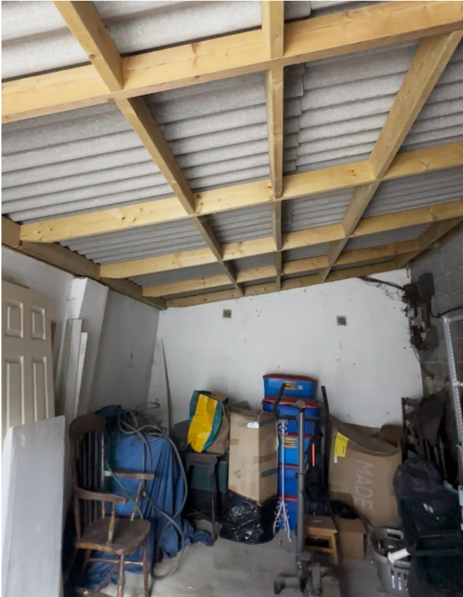
Figure 2; Photographs of showing the interior of the barn with roof rafters and asbestos sheets
