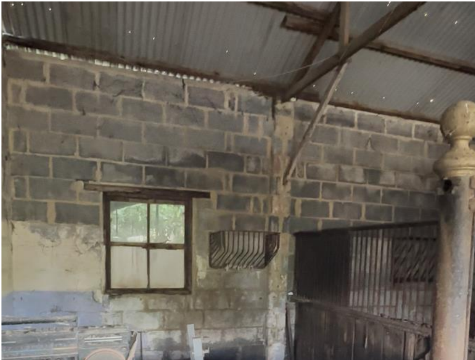
Figure 4; Photographs of showing the masonry piers with reinforcing piers
