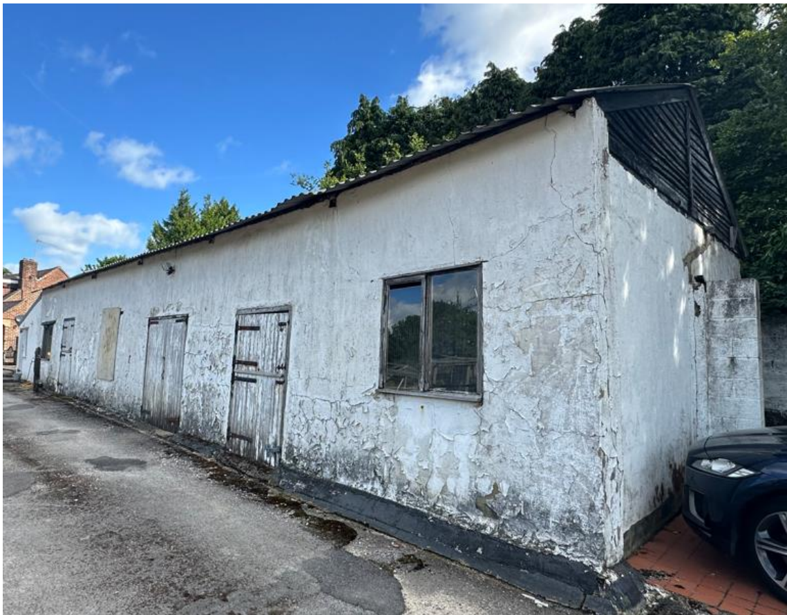
Figure 1. Photograph showing the exterior condition of the existing building
