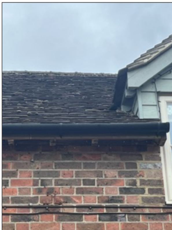
Photograph 2. (left) Area of loose tiles on dwelling around gable
