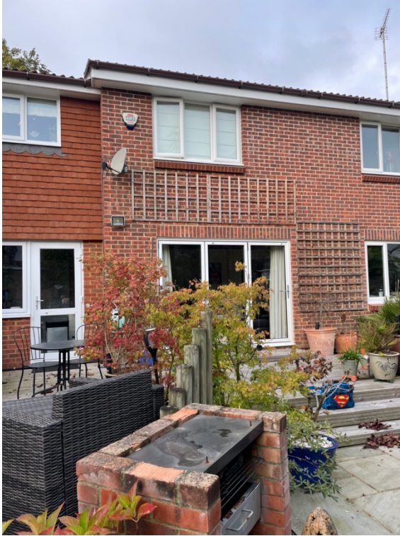
View looking west showing rear elevation
