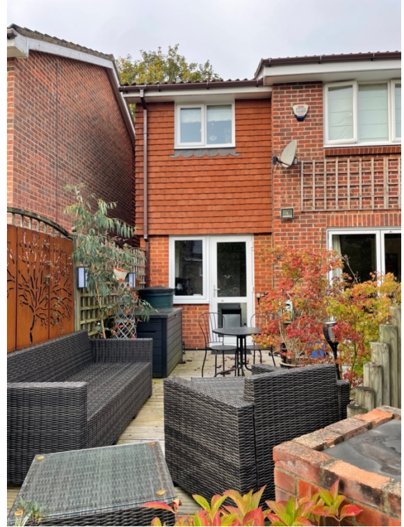
View looking west showing rear elevation
