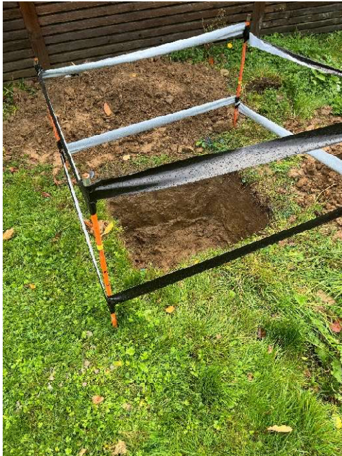
Soakaway Test Pit – Location
