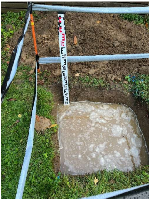
Soakaway Test Pit – Start Water Level 400mm
