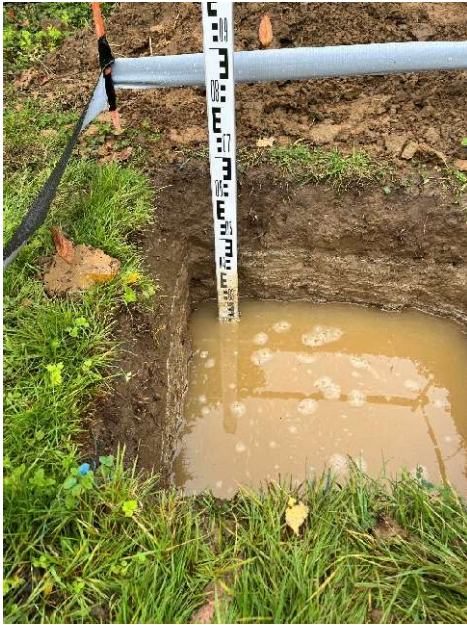
Soakaway Test Pit – Start Water Level 200mm
