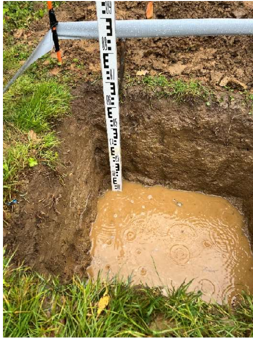
Soakaway Test Pit – Start Water Level 100mm
