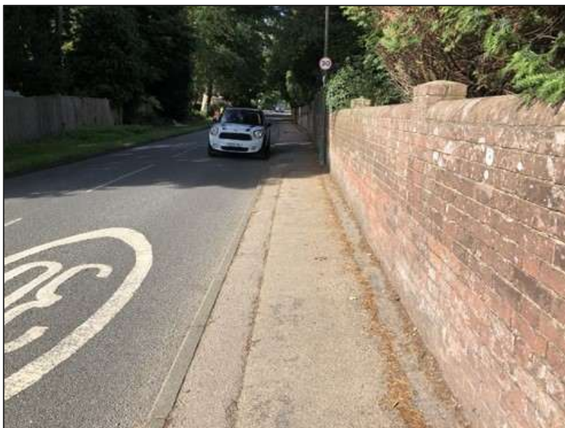
Figure 5.2: Pedestrian Footway on Borers Arms Road
