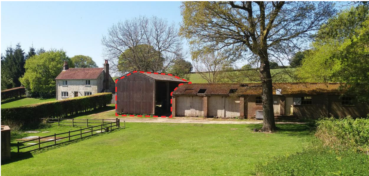
3.4.3 / i Existing Stables - Marked building has been demolished.
