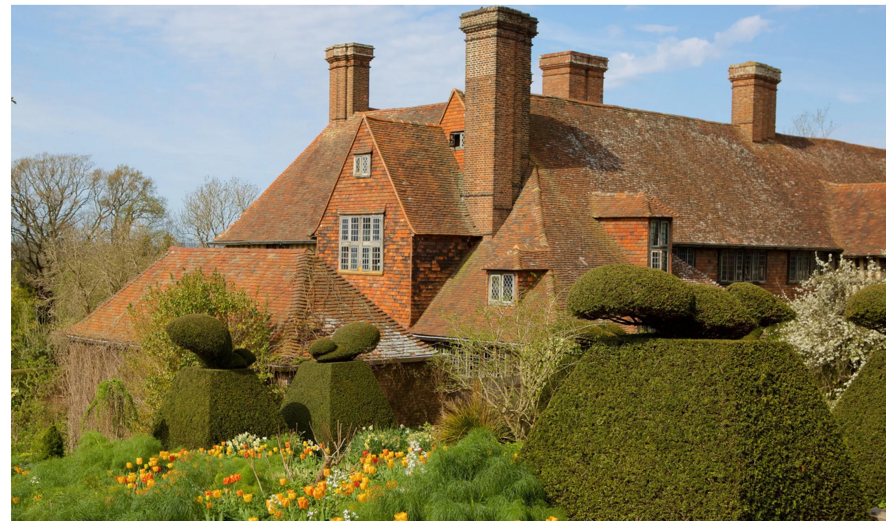
3.2.1 / ii Great Dixter (1910-12) where vertical hung tiles have been applied on the facade.
