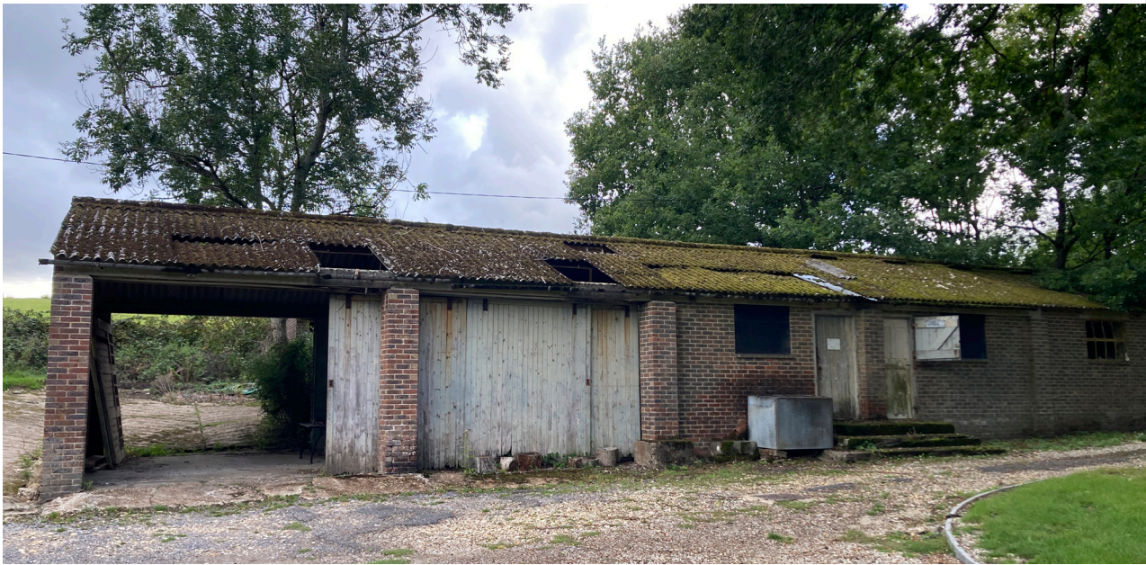
3.4 / i Existing Stables
