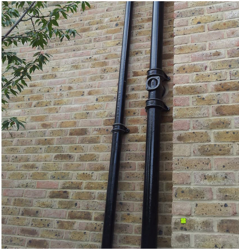
7 Cast iron gutter and rainpipe
