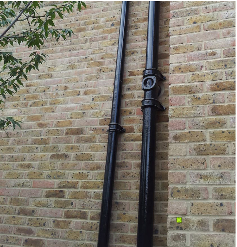
7 Cast iron gutter and rainpipe
