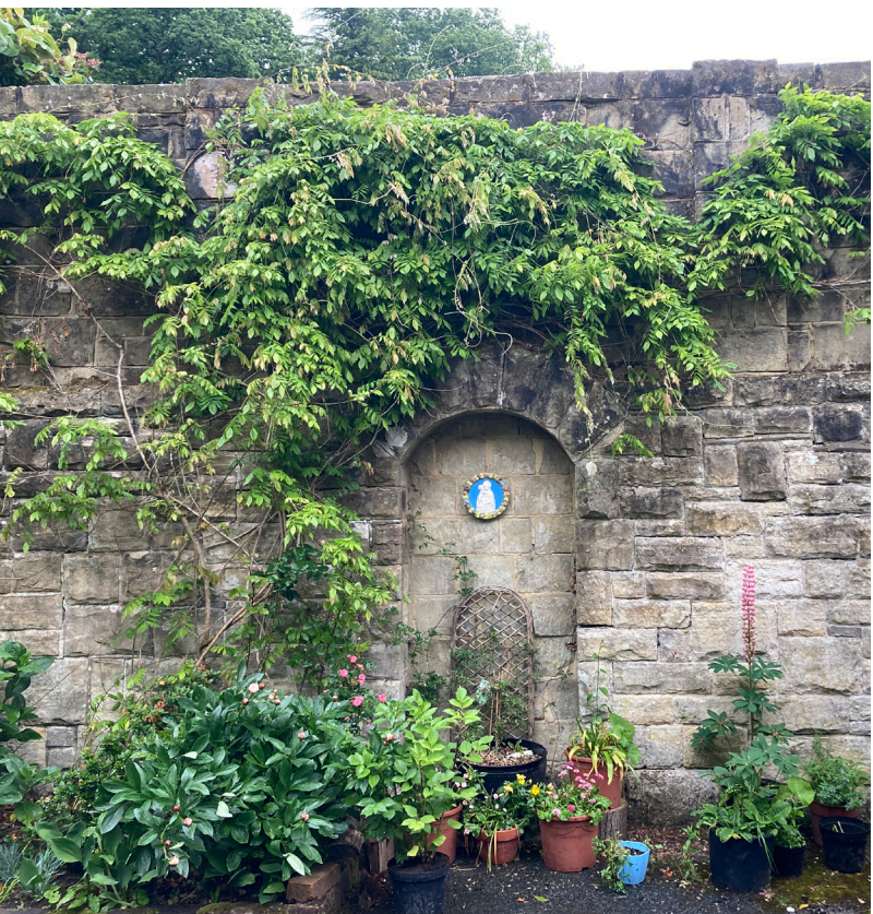
8 Existing sandstone to be carefully cleaned and salvaged from the on-site wall prior to demolition for reuse.
