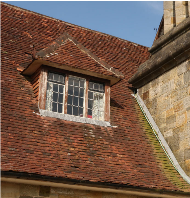
1 Reclaimed clay tiles to be blended with the existing roof to preserve its character
