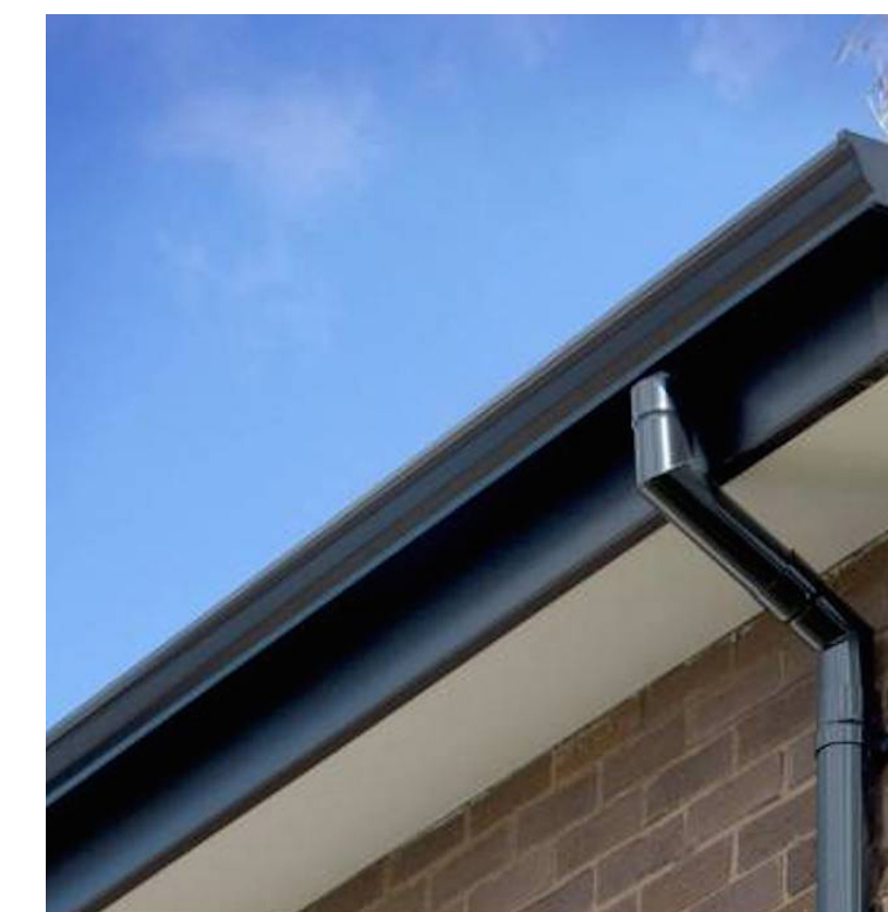
7 Aluminium Seamless Gutters Colour RAL 7034
