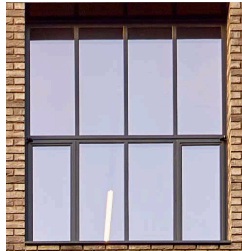
4 Steel (FerroFinestra W50 TB system) windows
