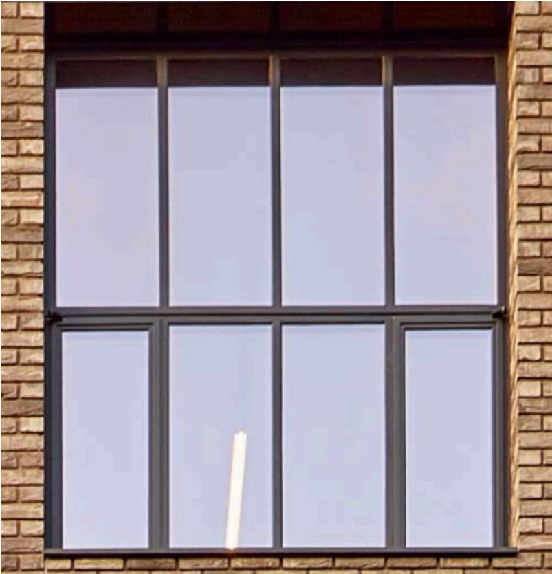
4 Steel (FerroFinestra W50 TB system) windows
