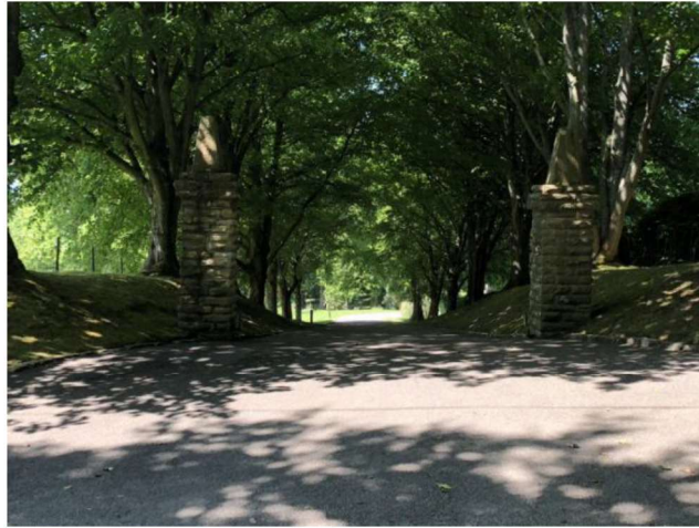
Photograph 3: Existing Main Vehicle Access
