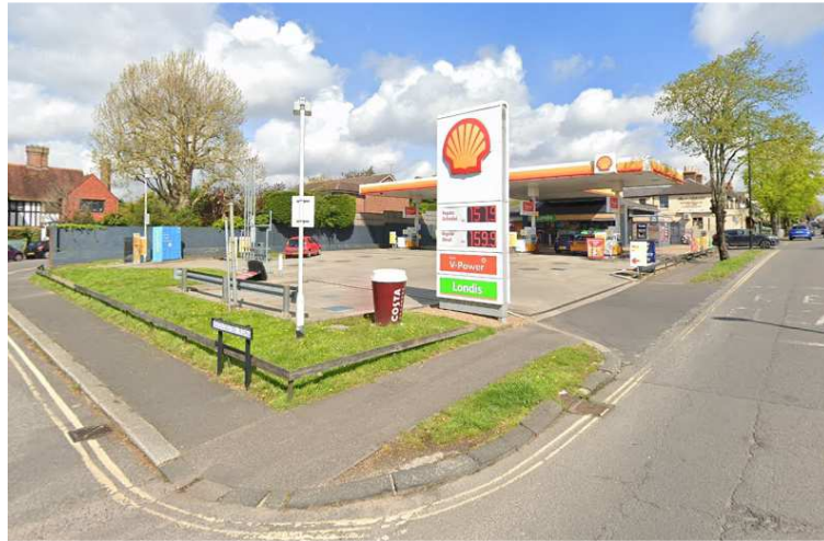
View from site entry point showing forecourt Shell canopy fascia and flag sign
