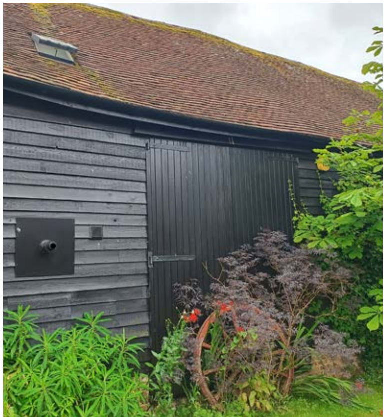
Current view of northern elevation
