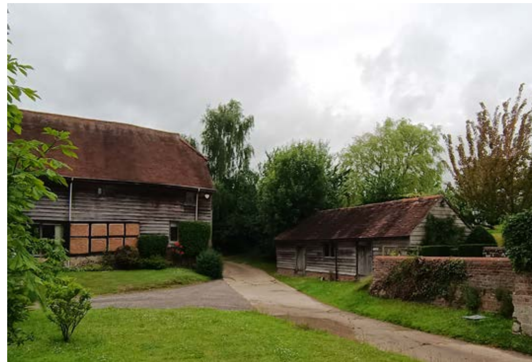
Neighbouring Barn clad in grey/silver timber
