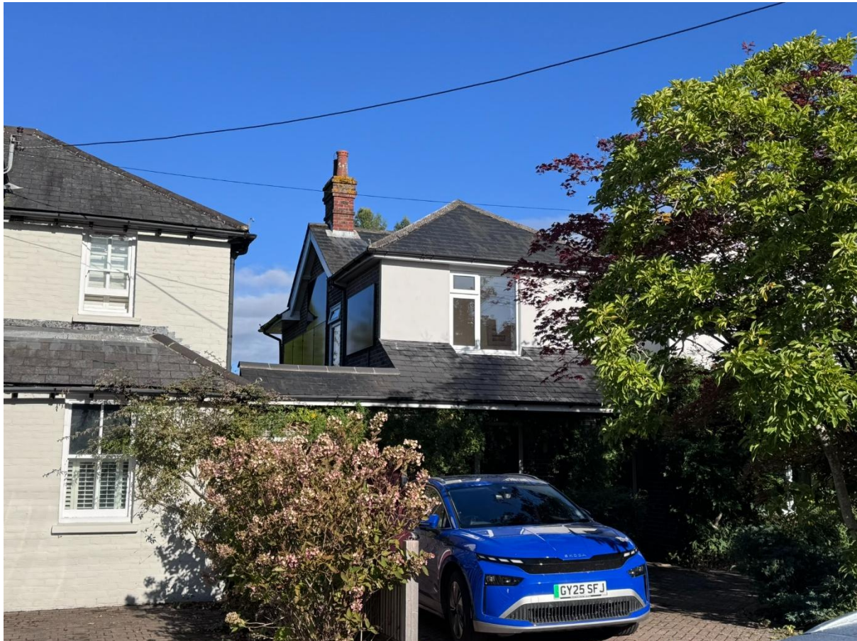
Figure 5: 6 SW facing solar panels on SW wall, viewed from Lewes Road
