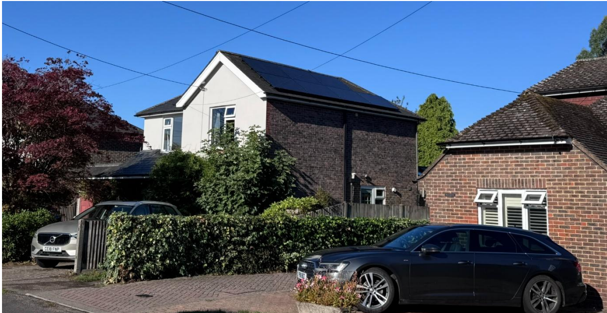
Figure 3: 7 NE facing solar panels on 35° pitch slate roof, viewed from Lewes Road
