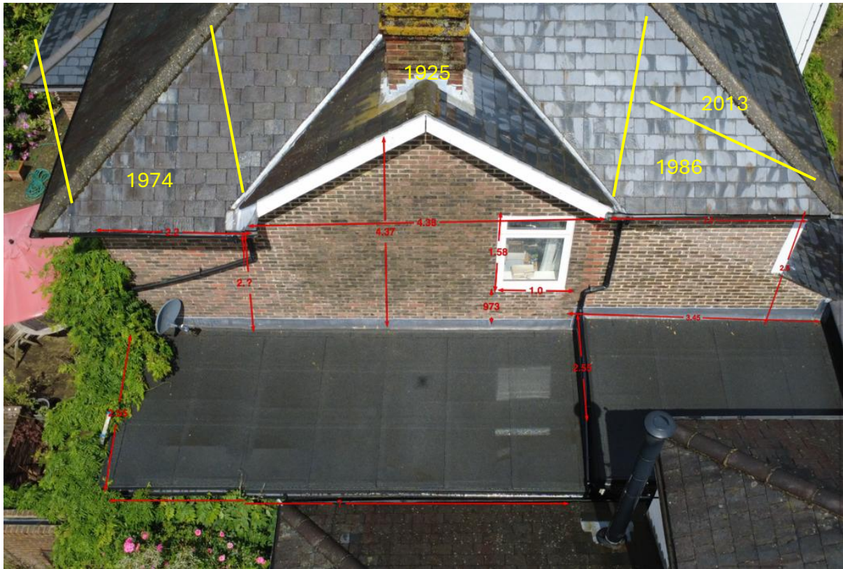
Figure 8: SW wall showing mix of brickwork revealing 4 phases of construction, now concealed by solar panels
