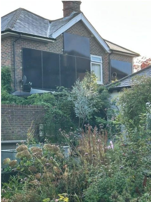
Figure 6: View from Hamsey Cottage garden - Image 1
