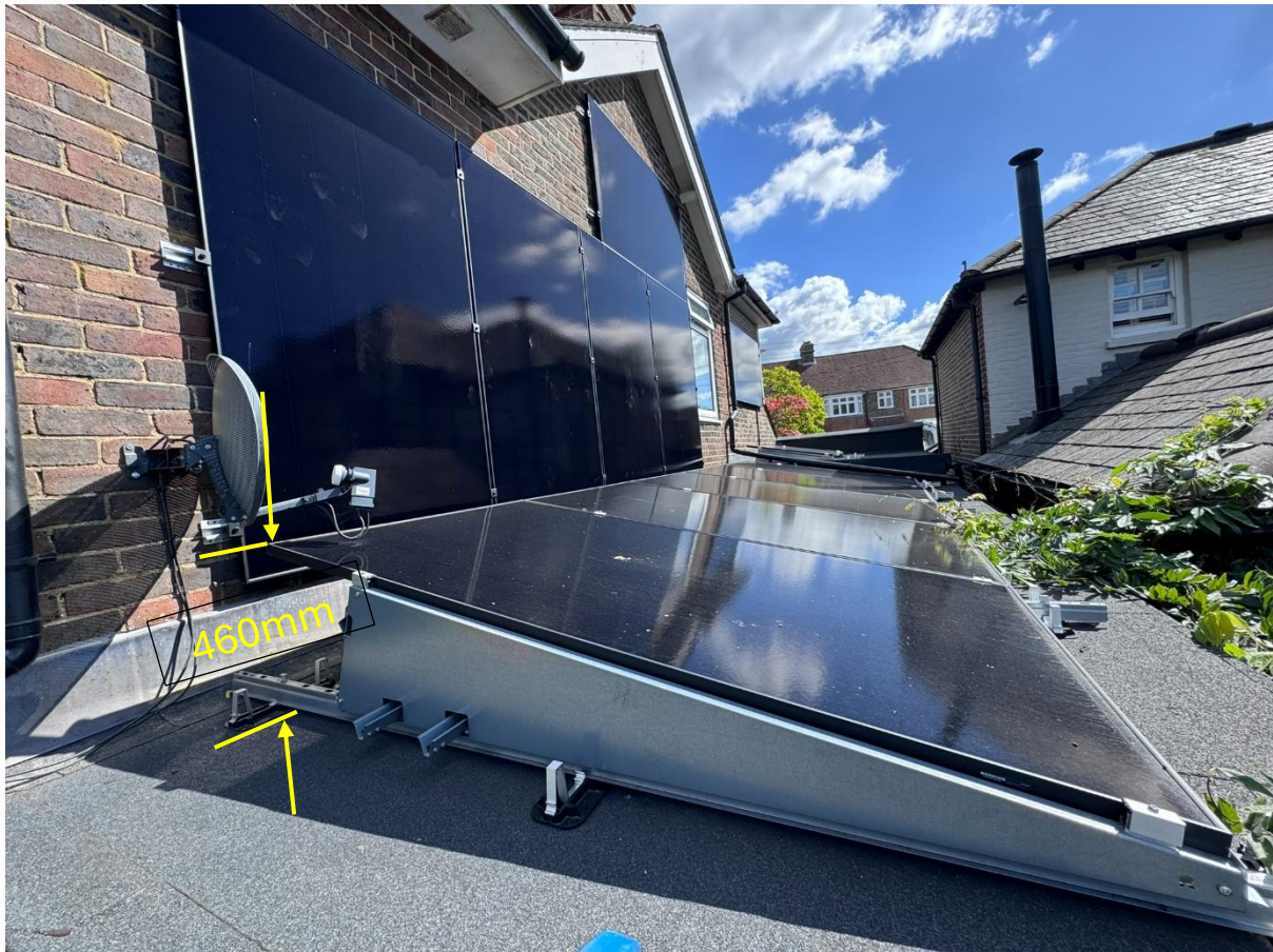
Figure 2: Black bifacial panels with black frames on Van der Valk mounting system – maximum 460mm upstand
