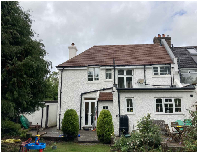
Photo 3: Existing rear elevation
