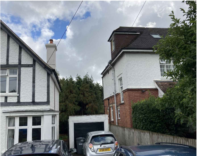
Photo 2: Existing front / side view
