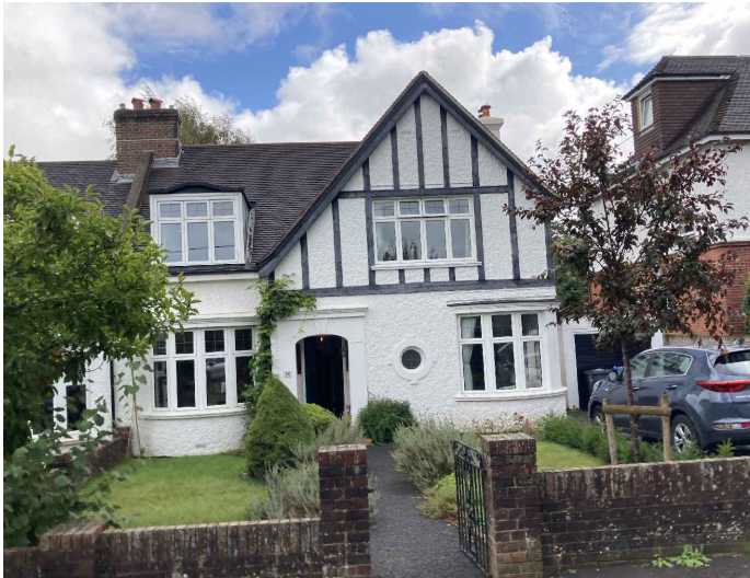
Photo 1: Existing front elevation
