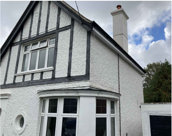
Photo 4: Existing front / side view
