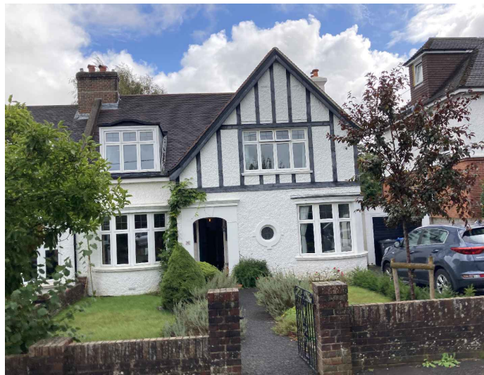
Photo 1: Existing front elevation
