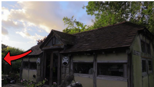
Photograph 2. Emergence of two common pipistrelles from gaps under roof tiles on the annexe at 19 and 28 minutes after sunset (Roost 2).
