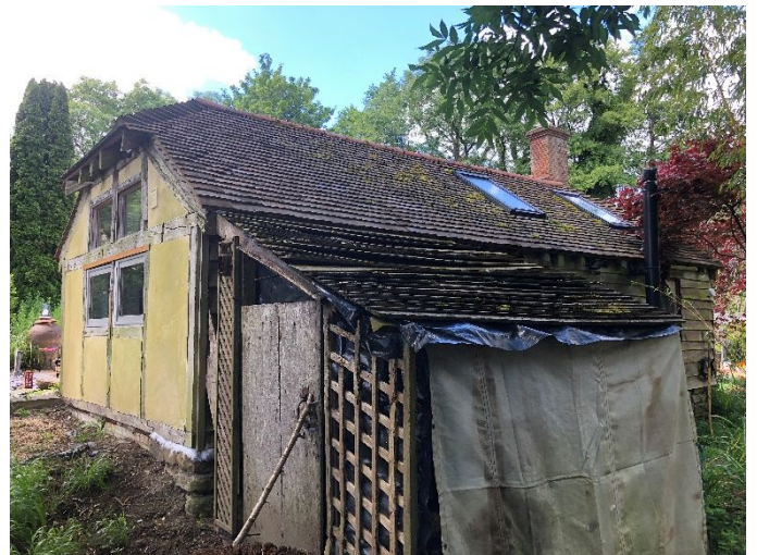
Photograph 6. Northern and eastern elevations of the annexe.
