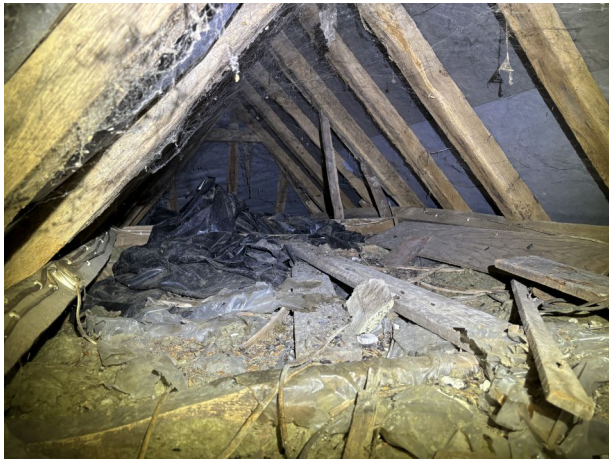
Photograph 1. The inaccessible section of the roof void within the property.
