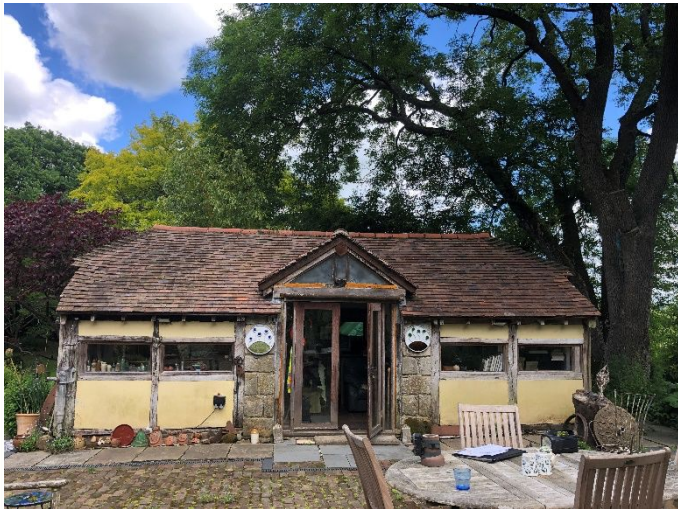
Photograph 3. Southern elevation of the annexe.
