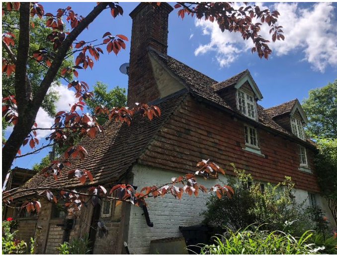
Photograph 1. Northern and western elevations of the property.
