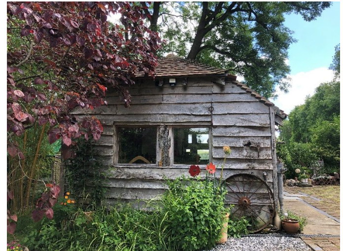
Photograph 4. Western elevation of the annexe.
