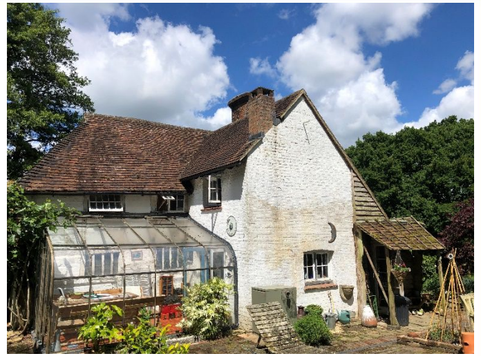
Photograph 2. Southern and eastern elevations of the property.
