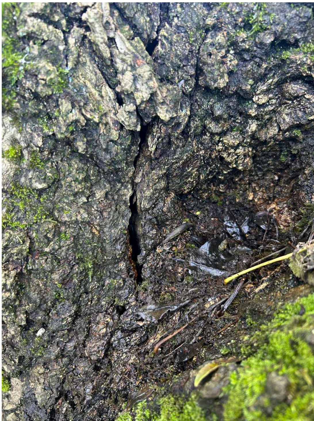
T1 – Basal crack, close-up
