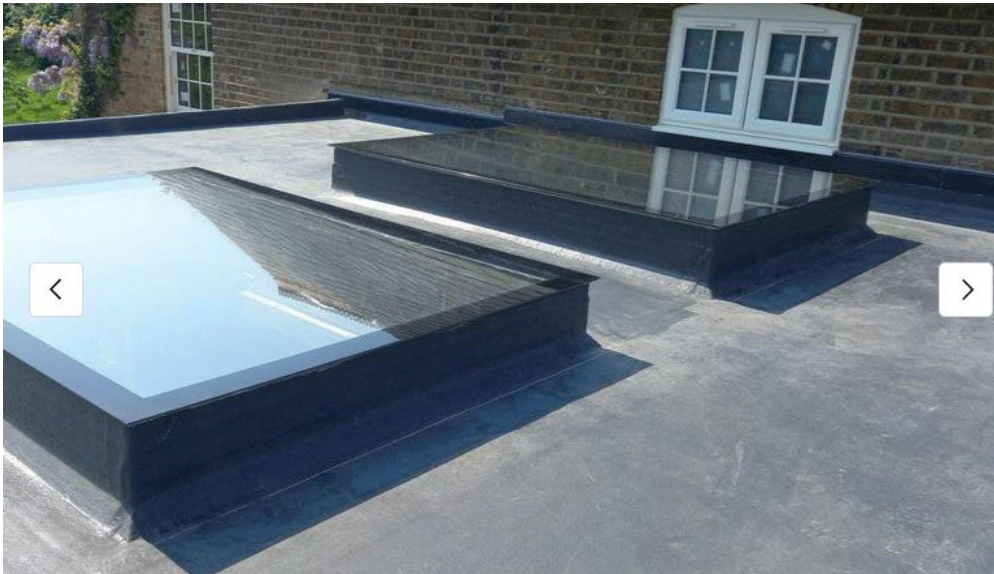
Roof and rooflight Single ply roof membrane with low profile, aluminum framed glazed roof lights
