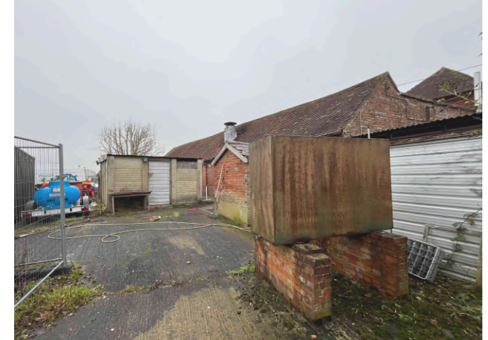
West Elevation viewed from the south
