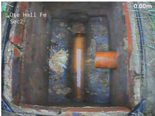
1, 00:00:00, 0.00 m Start node, manhole, reference: FW4
