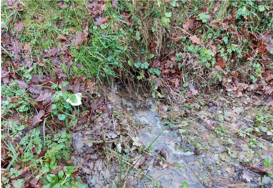
Photo 3: Culvert outlet from receiving ditch entering ditch on opposite side of access road, viewed from the east
