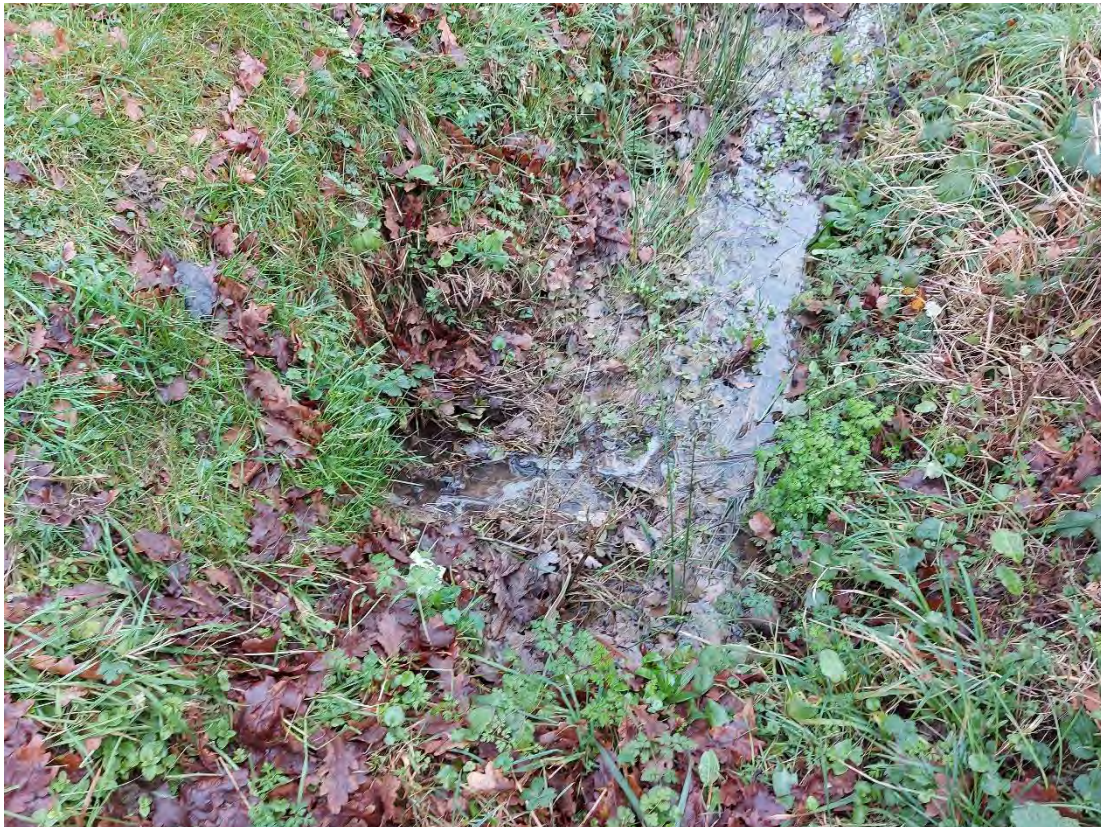
Photo 4: Culvert outlet from receiving ditch entering ditch on opposite side of access road, viewed from the south
