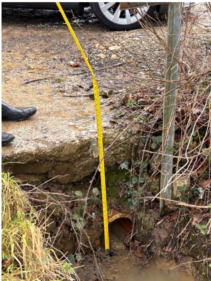
Photos 5 and 6: Measurements of existing culverts showing 225mm diameter
