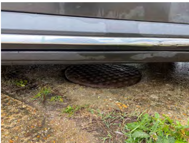
Foul Sewer chamber location
