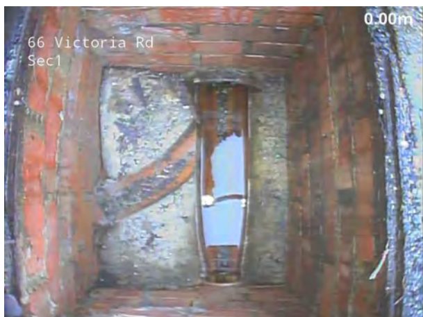
1, 00:00:00, 0.00 m Start node, manhole, reference: SW2
