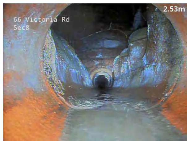
2, 00:00:31, 2.80 m Finish node, manhole, reference: FW1
