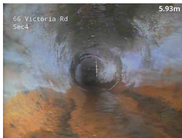
8, 00:00:55, 6.00 m Settled deposits, coarse, 15% cross-sectional area loss, finish
