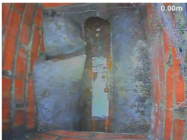
1, 00:00:00, 0.00 m Start node, manhole, reference: SW1
