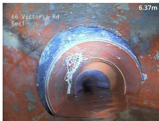
10, 00:01:21, 6.50 m Pipe material changes to polyvinyl chloride at this point
