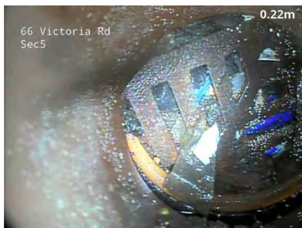
3, 00:00:15, 0.40 m Survey abandoned, Unable to continue
