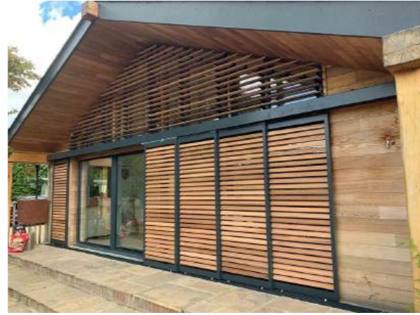
Example of Timber Brise Soleil
