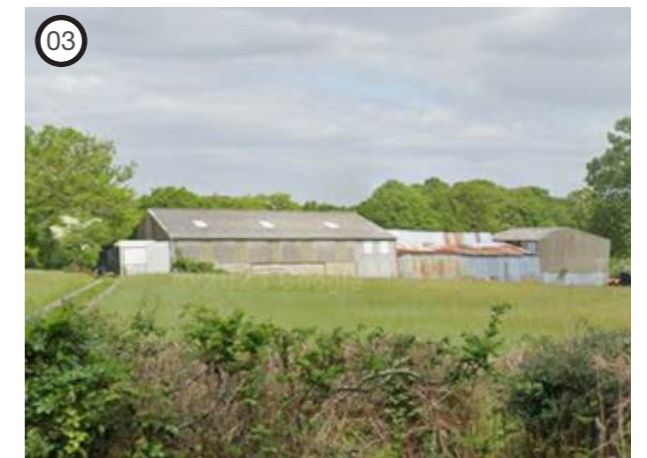
Farmhouses adjacent to the site
