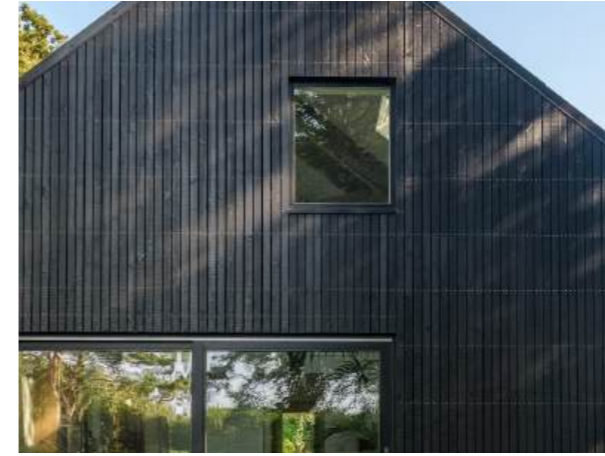
Example of charred timber cladding
