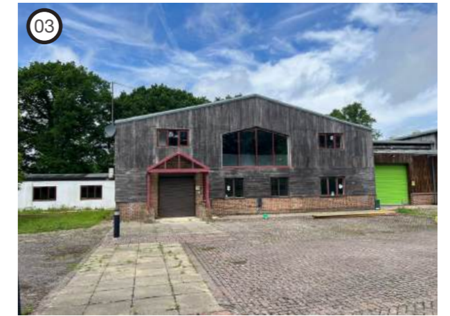
Existing Building front elevation
