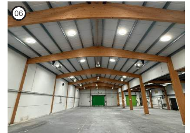
Interior of building A, Glulam structure
