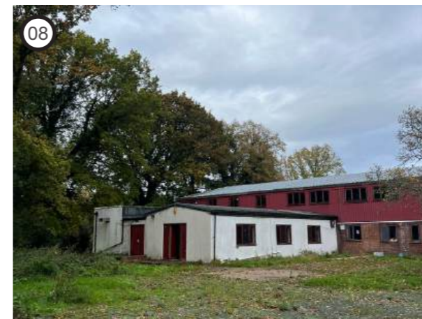
Existing extension (to be demolished)
