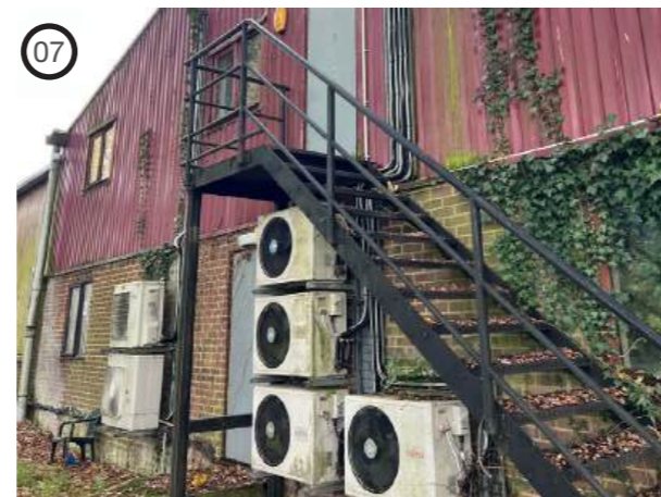
Existing fire escape stair to the rear of the building
