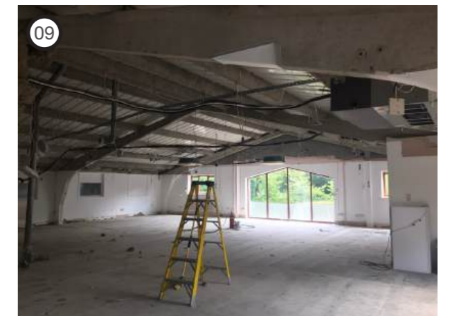
Interior of building B mezzanine level, concrete structure
