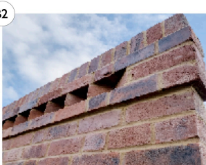
1.2M BRICK BOUNDARY WALL
