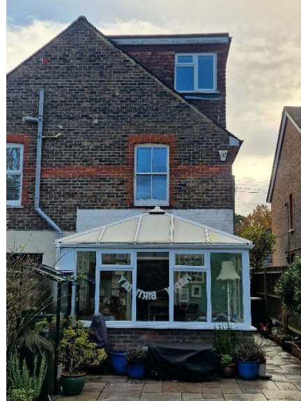
Rear Elevation (showing conservatory to be demolished)
