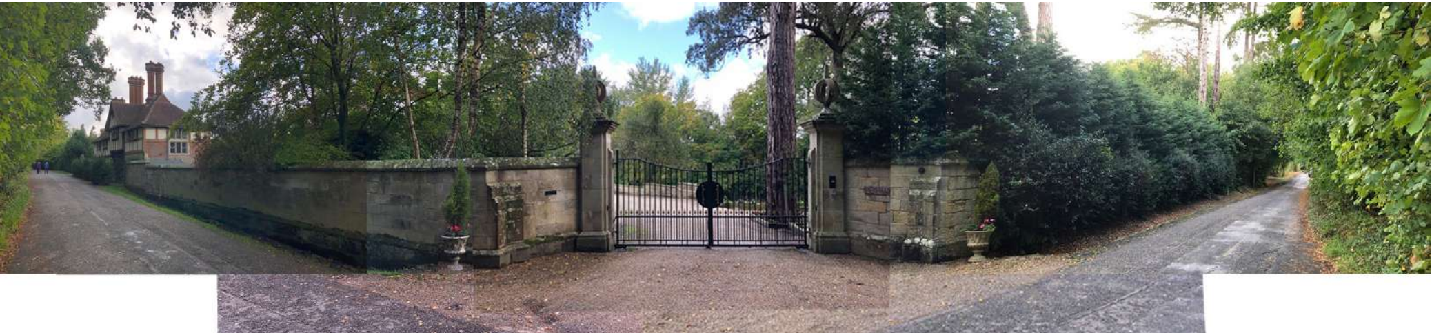
A03 - Looking West towards main entrance to site (see 11 on site plan) from Chownes Mead Lane with Coach House to left of frame
