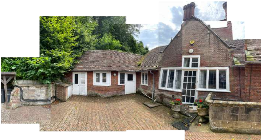
B04 - Rear of Chownes Mead looking South
