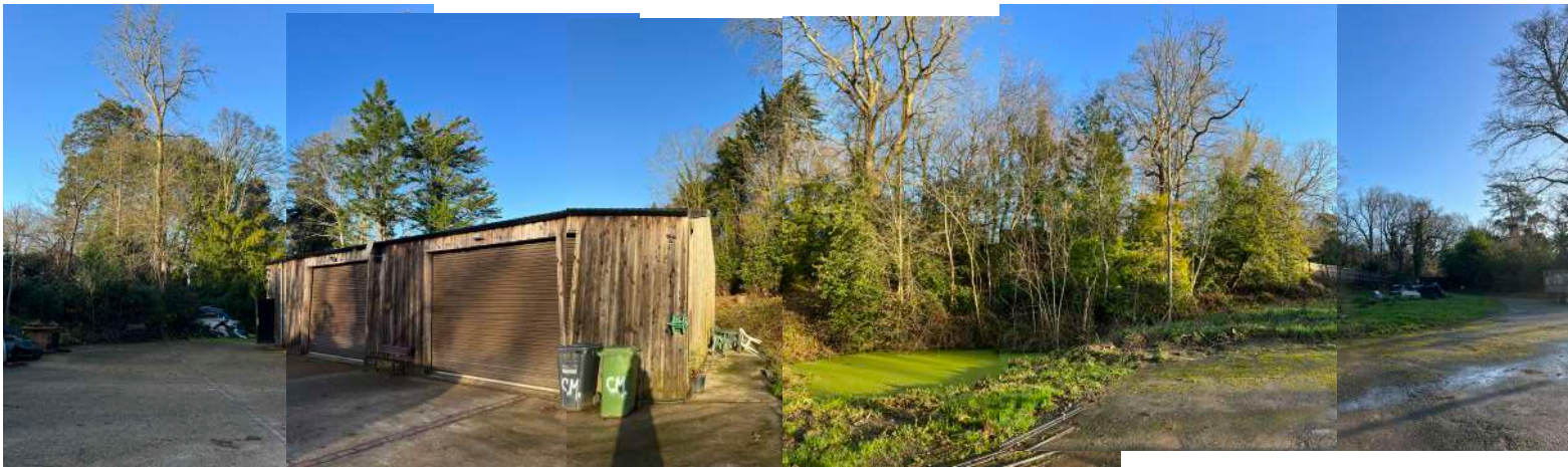
F06- Area of hardstanding to South of barn
