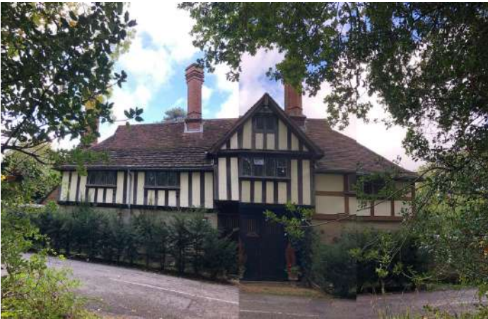
A01 - Looking West towards the Coach House from Chownes Mead Lane
