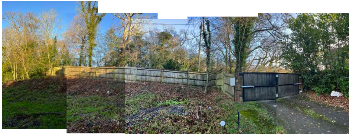
F02- Area of proposed new entrance to left of existing entrance
