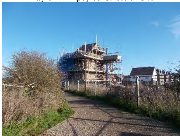
Taylor Wimpey construction site
