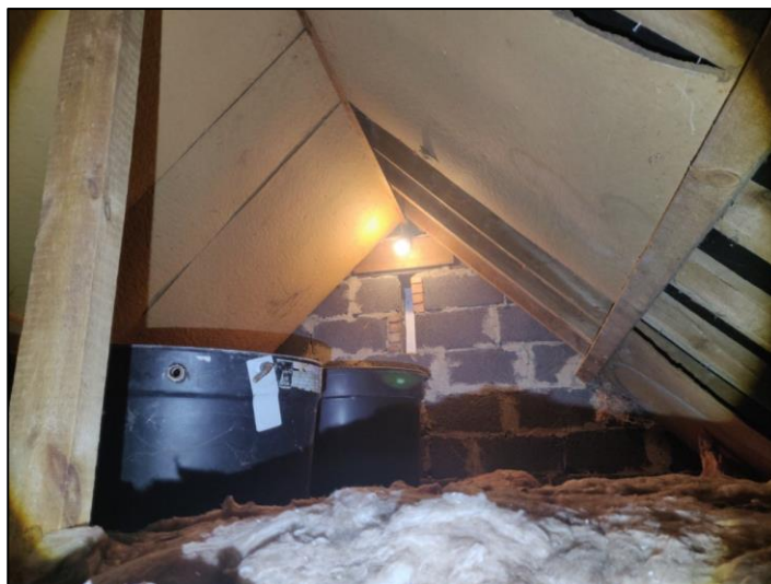
Photo 4.8: Internal roof void of building B1a, facing west.
