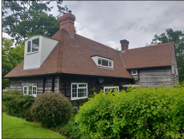
Photo 4.6: South-western aspect of building B1a.
