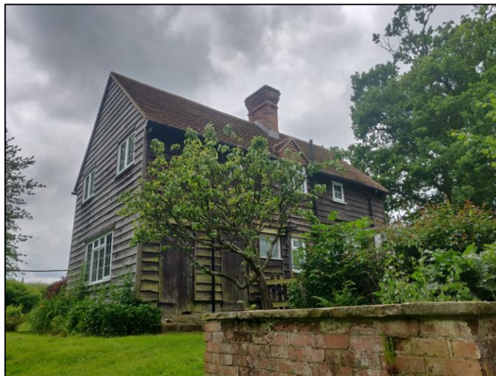
Photo 4.7: South-eastern aspect of building B1a.
