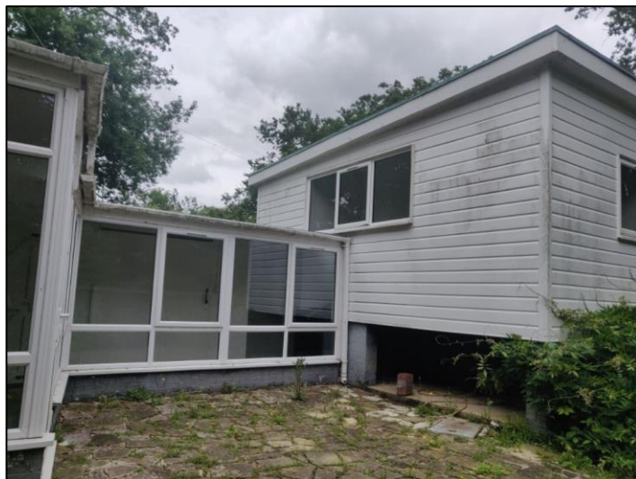
Photo 4.10: Walkway that joins buildings B1a and B1b.
