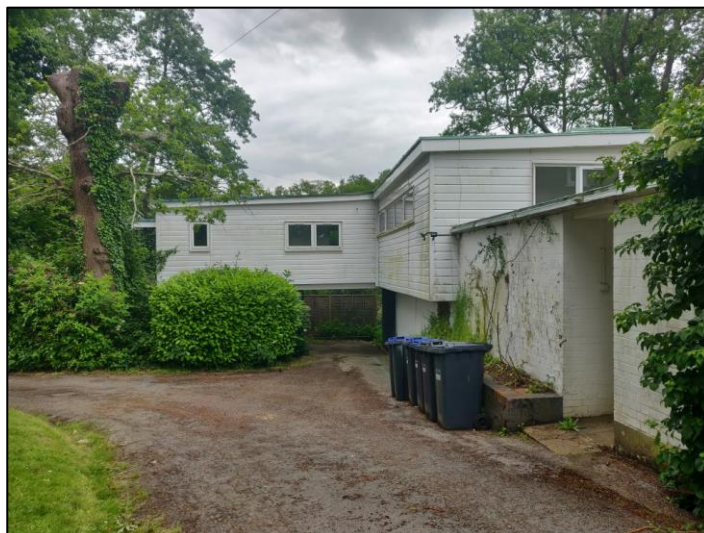
Photo 4.11: North-western aspects of building B1b.
