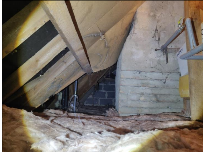
Photo 4.9: Internal roof void of building B1a, facing east.
