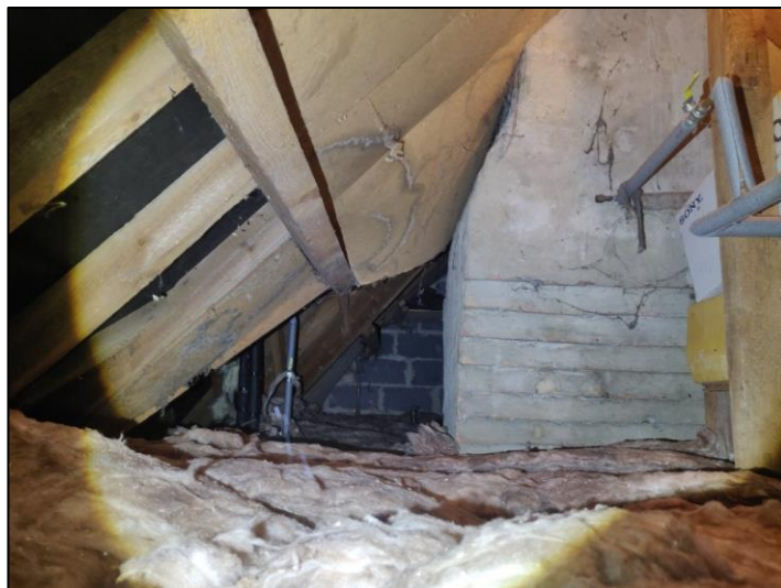
Photo 4.7: Internal roof void of building B1a, facing east.
