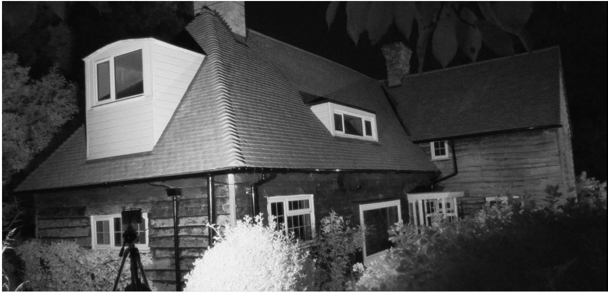
Photo A3.1: Canon IR image at the darkest point of the survey facing the south-western aspect of the building, 26 th June 2024.
