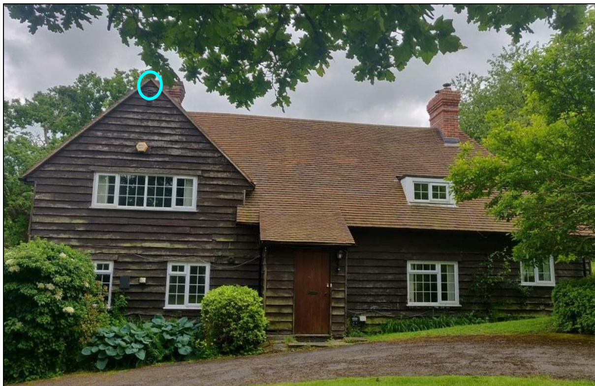
Photo A3.6: Common pipistrelle bat emergence locations during the first survey (26 th June 2024) and third survey (7 th August 2024) circled in blue, on the northern aspect of building B1a.
