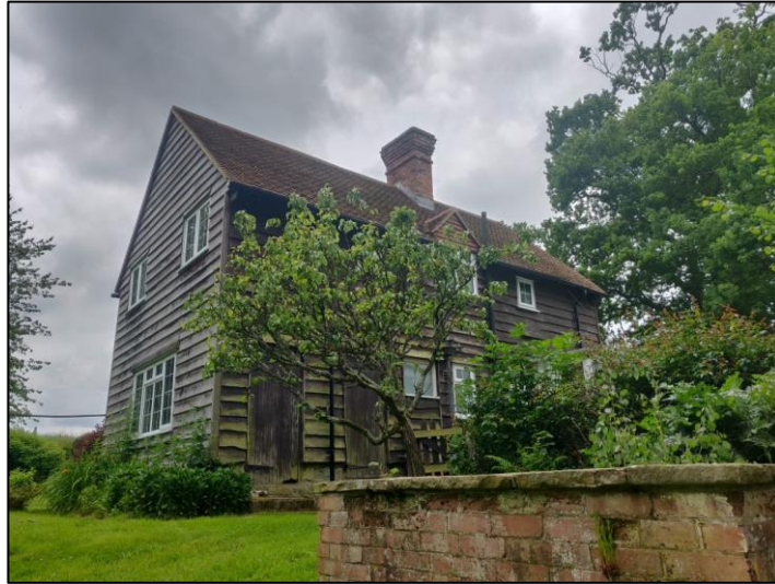
Photo 4.5: South-eastern aspect of building B1a.
