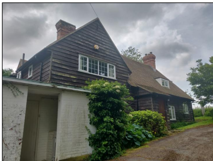
Photo 4.1: North-eastern aspect of building B1a.
