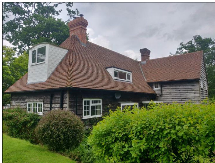
Photo 4.4: South-western aspect of building B1a.
