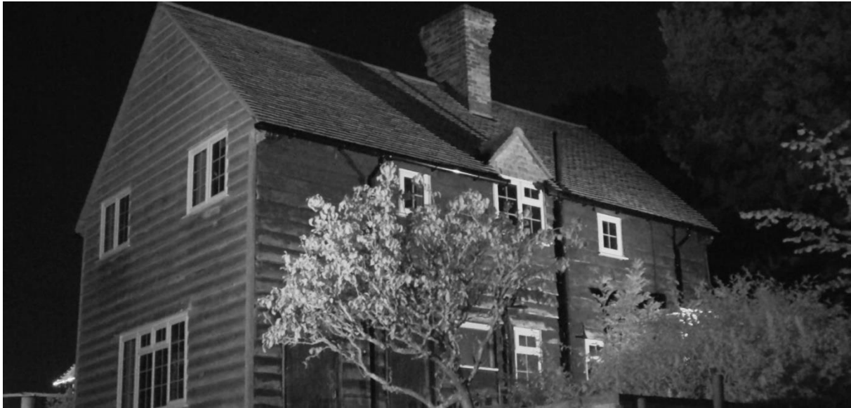
Photo A3.3: Canon IR image at the darkest point of the survey facing the southeastern aspect of the building, 26 th June 2024.
