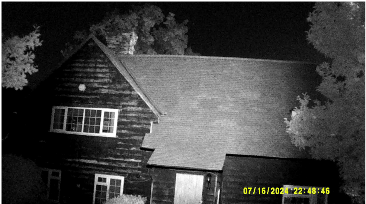
Photo A3.2: Nightfox IR image at the darkest point of the survey facing the northern aspect of the building, 16 th July 2024.
