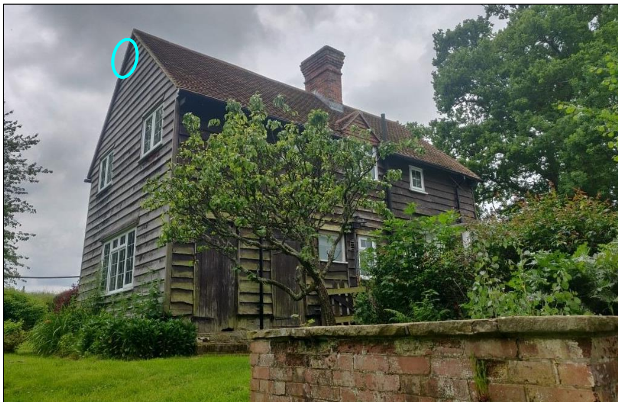
Photo A3.5: Common pipistrelle bat emergence location during the third survey (7 th August 2024) circled in blue, on the southeastern aspect of building B1a.
