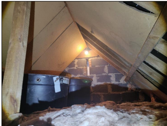
Photo 4.6: Internal roof void of building B1a, facing west.
