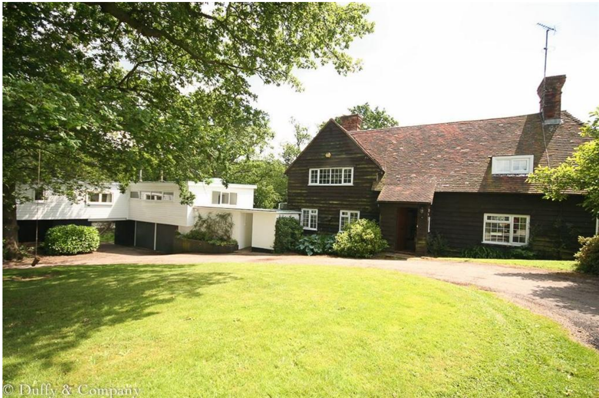
Photo of The Lake House from the north
