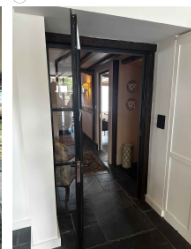
New crittall style door between existing dwelling and new extension
