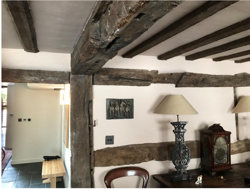
Figure 12: main E-W ceiling beam to the living room showing the location of an original partition and doorway adjacent to the northwest wall. The timber jamb post is proposed to be reinstated.
