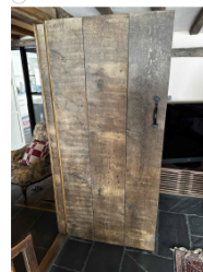
New timber plank door
