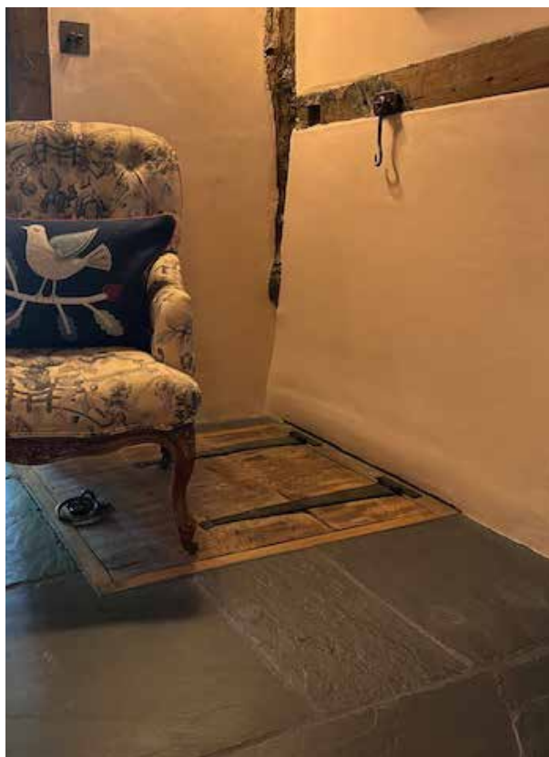
Ground Floor -access hatch to basement
