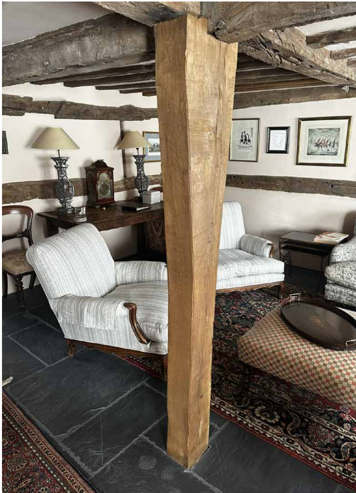
Ground Floor - steel post replaced with timber post
