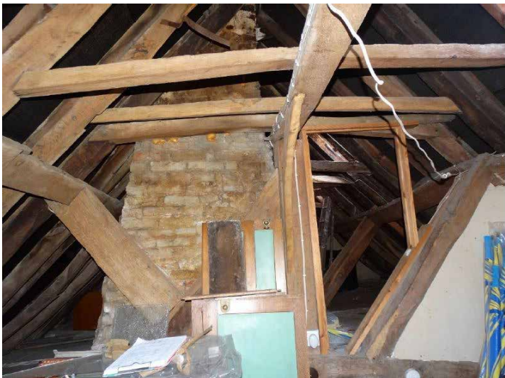
Attic, chimney stack in the background
