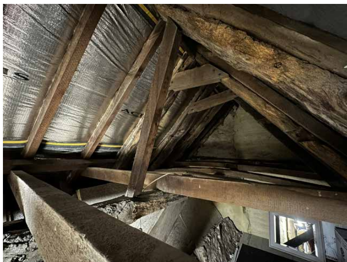
Attic - historic timber frame roof
