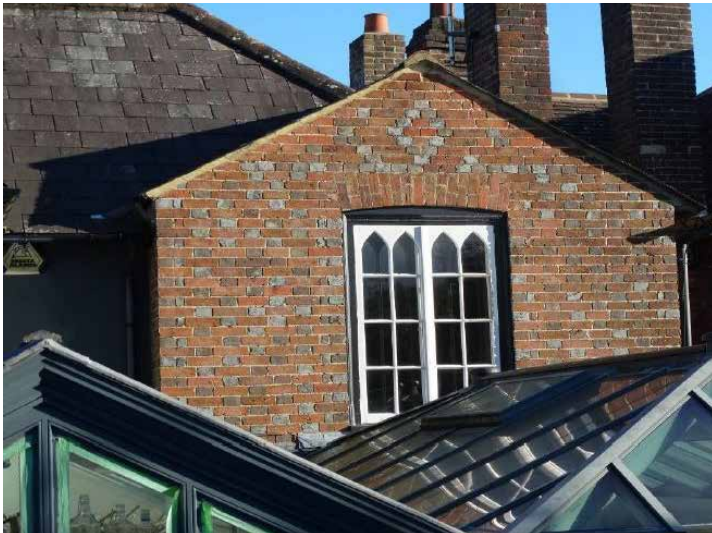
Historic rear extension with gothic window
