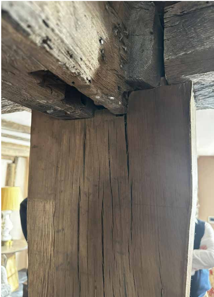
Ground Floor - steel post replaced with timber gunstock post
