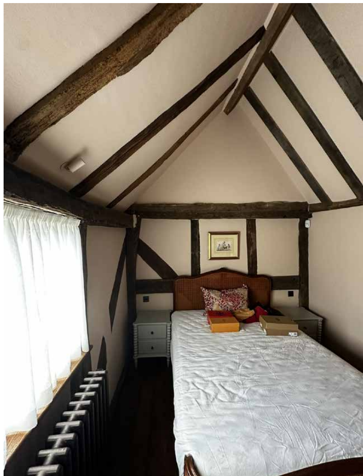
First Floor - historic timber frame roof
