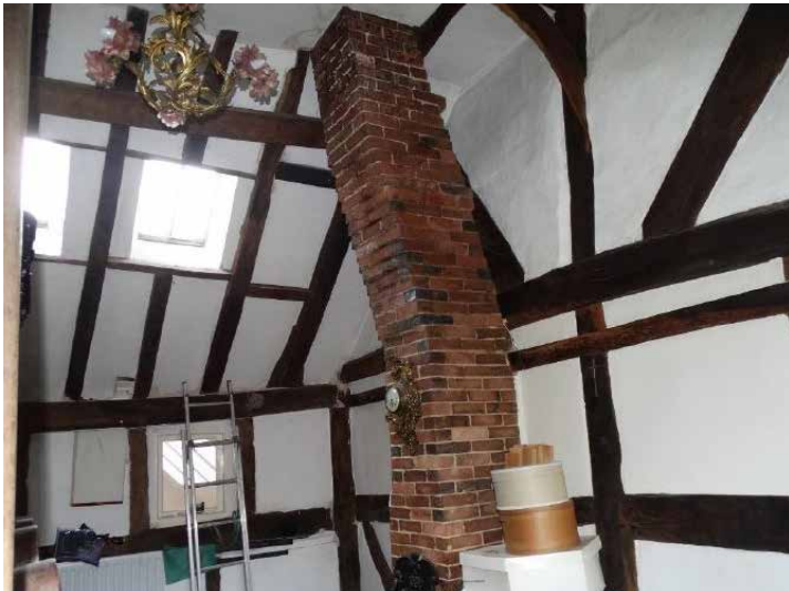
First floor bedroom, chimney stack
