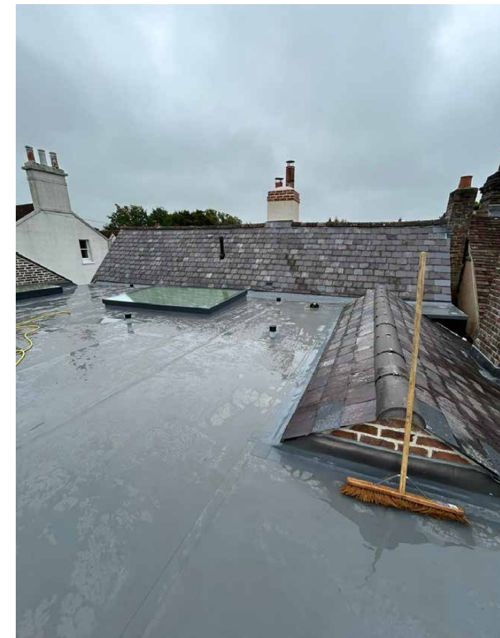
Roof - ridge of the historic extension above new flat roof
