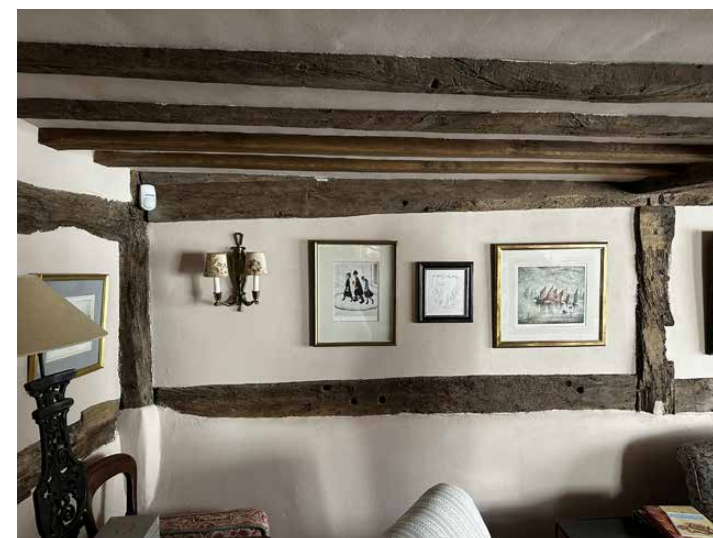
Historic timber frame wall, living room
