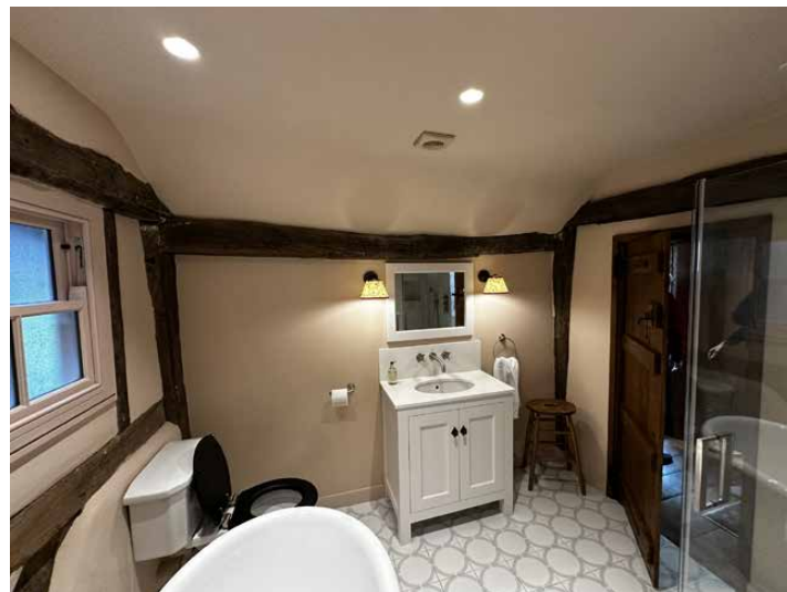
First Floor - bathroom
