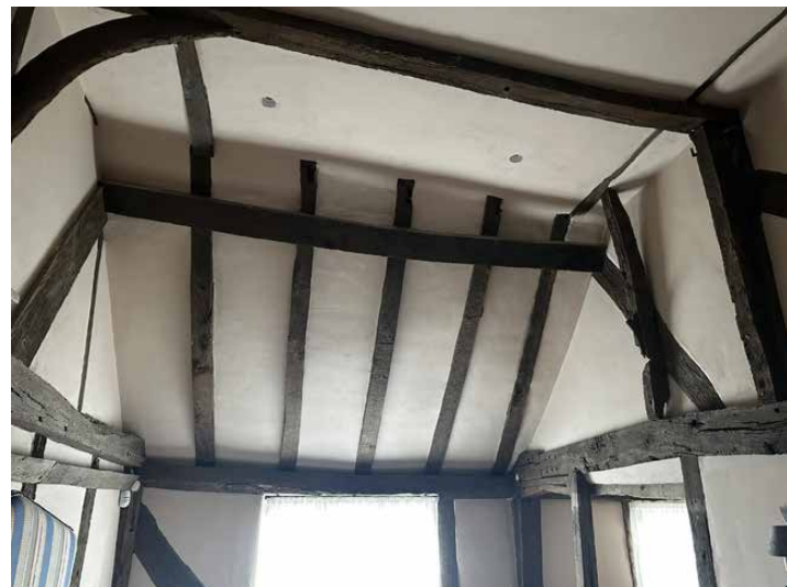
First Floor - historic timber frame roof
