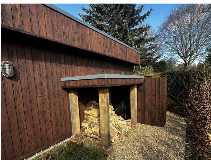
Covered loggery and irrigation tank enclosure adjacent to the garage
