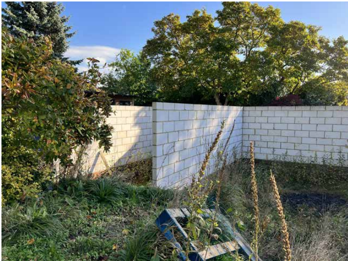
Garage walls constructed
