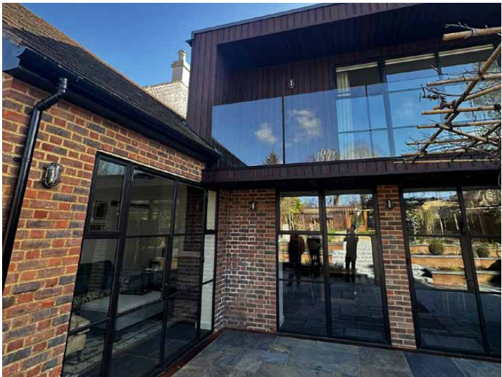
Rear elevation & re-constructed bake house
