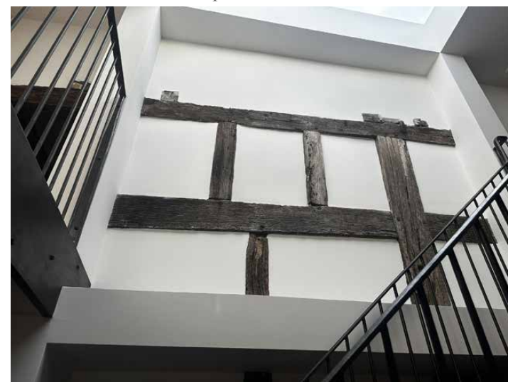
Historic timber frame wall in stairwell
