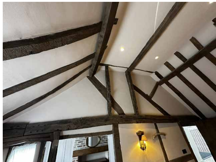
First Floor - historic timber frame roof
