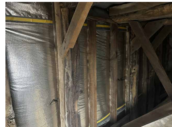
Attic - historic timber frame roof, new insulation
