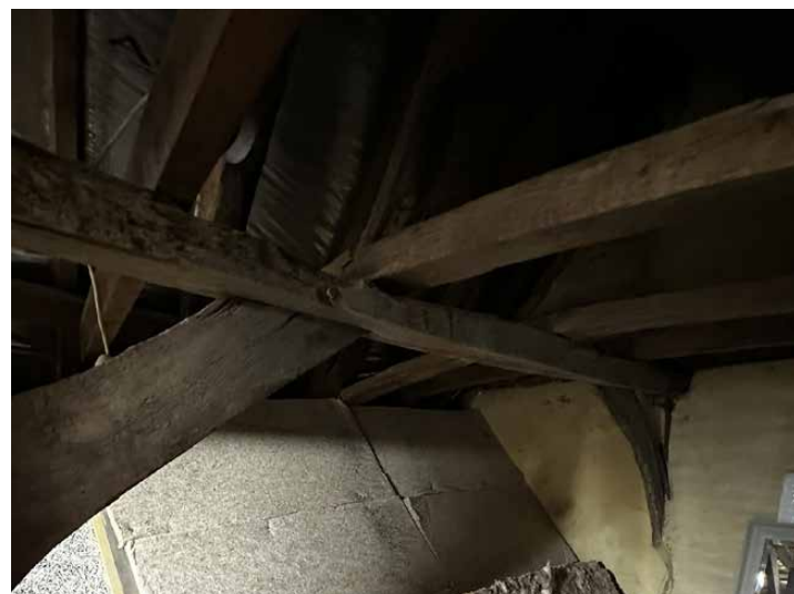
Attic - historic timber frame roof
