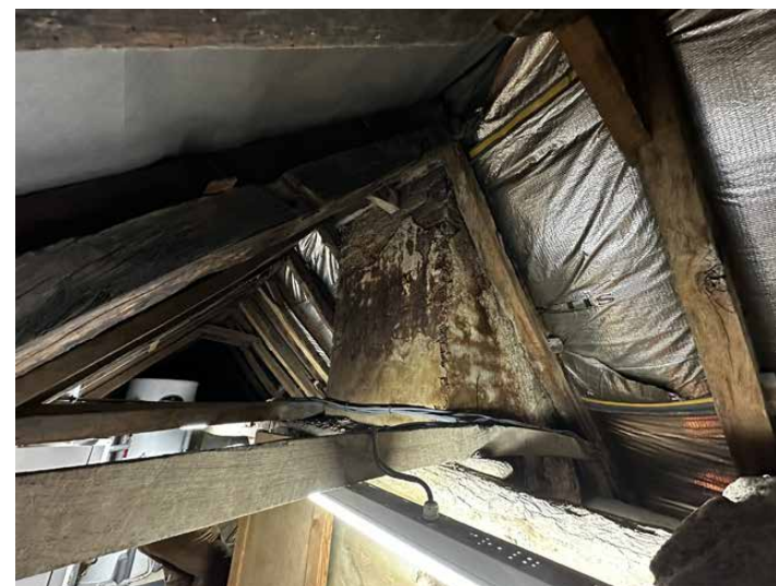
Attic - historic timber frame roof
