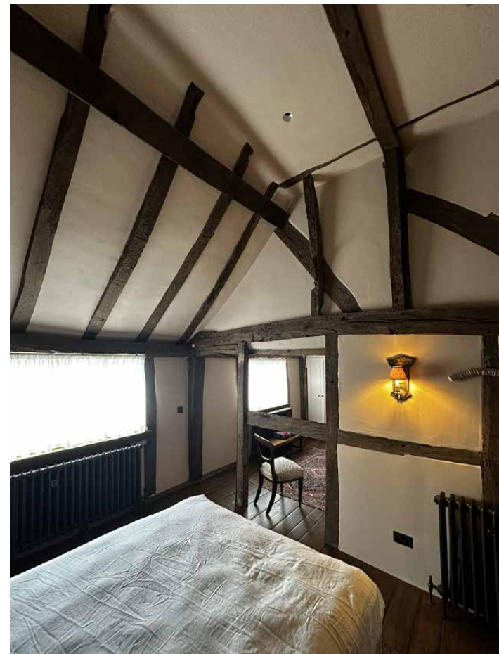
First Floor - historic timber frame roof
