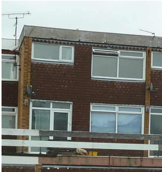
103 Church Walk, showing likely bathroom on left hand side of second floor and entrance corridor on left hand side of first floor
