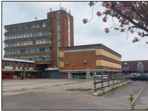
Figure 1: Boarded up building
