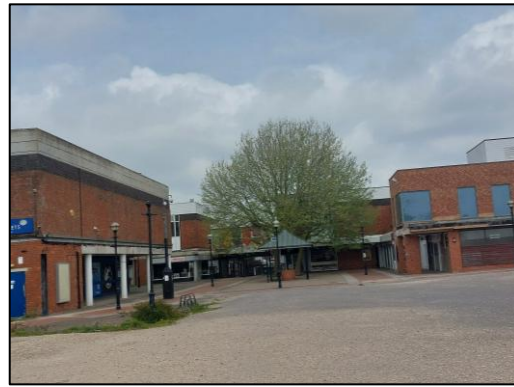
Figure 2: Central courtyard with boarded up buildings
