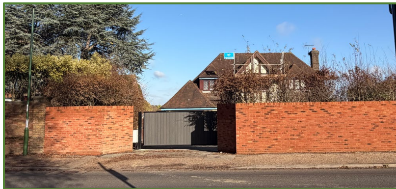
Photograph 2 – Brick wall as constructed
