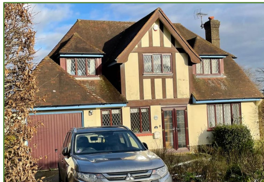
Photograph 1 – Front elevation of 50 Hurst Road
