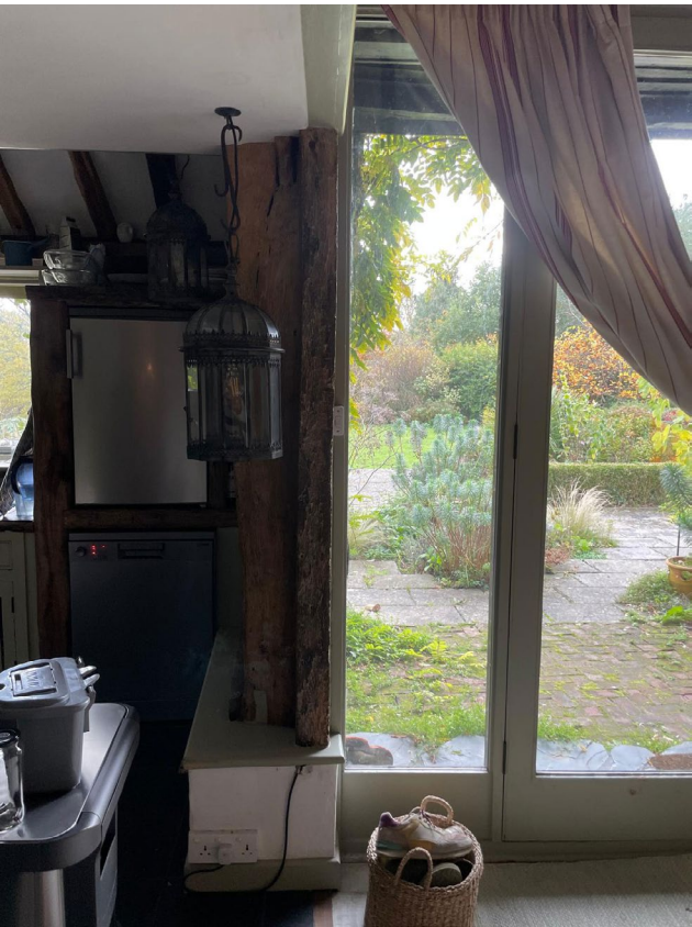
PHOTO C Two sides of original post are visible with a modern timber fixed in front forming door opening
