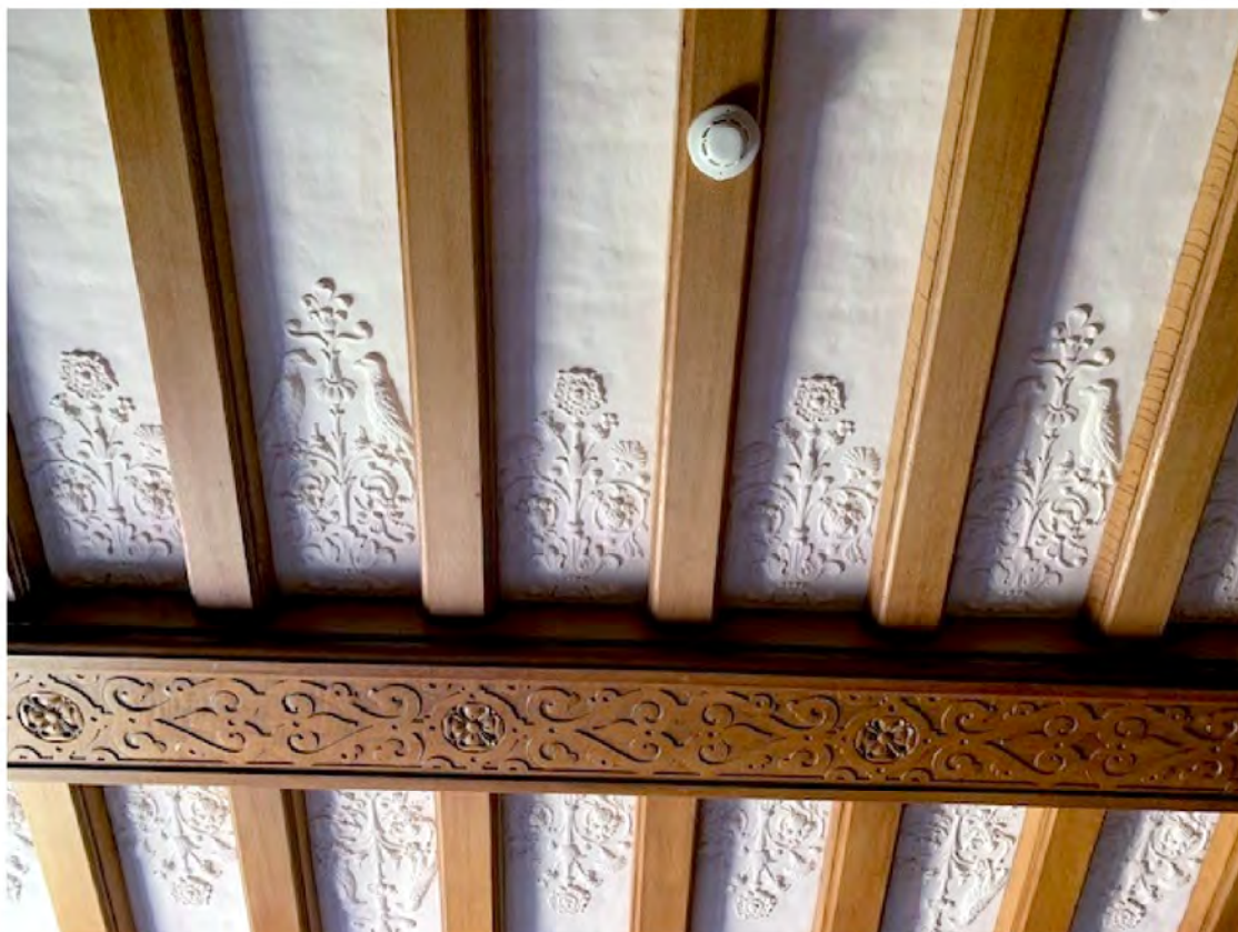
Plate 9: Study detail of ceiling
