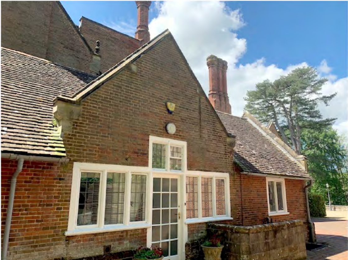
Plate 39: Northeast Elevation in service yard
