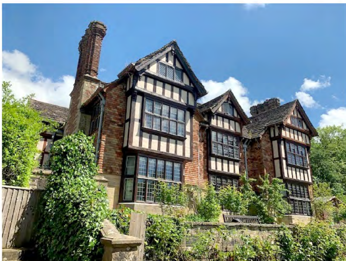
Plate 30: Southwest elevation viewed from level below terrace
