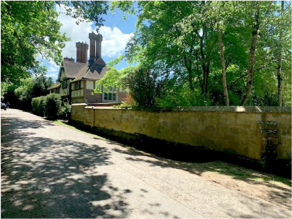
Plate 43: Chownes Mead Lane looking southeast towards The Lodge
