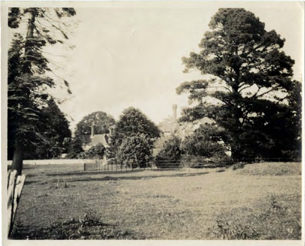
Plate 49: Archive Image sent of works to Gertrude Jekyll - northwest elevation from west
