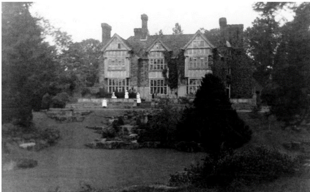
Plate 45: Archive Image of southwest elevation c.1943
