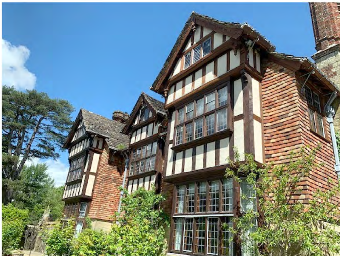
Plate 23: Southwest elevation from terrace
