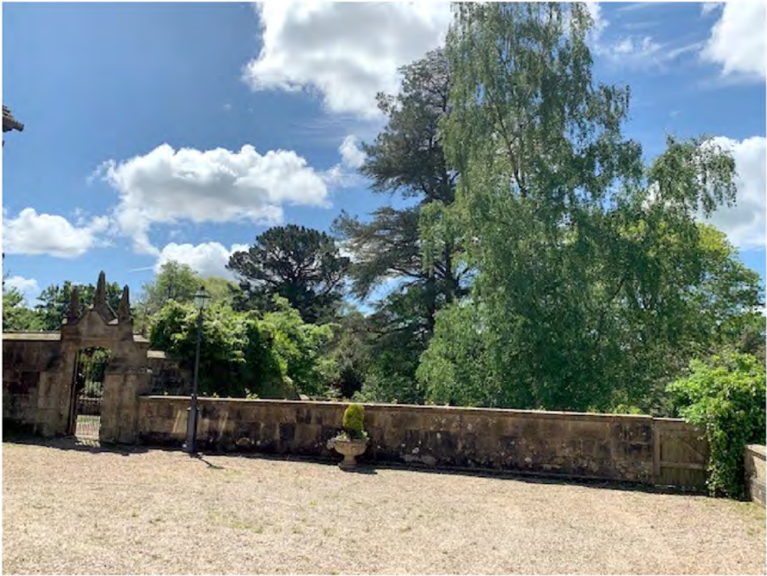
Plate 35: Garden wall to northwest terrace with inset gate detail
