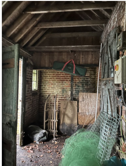
IM02 - Internal view looking south
