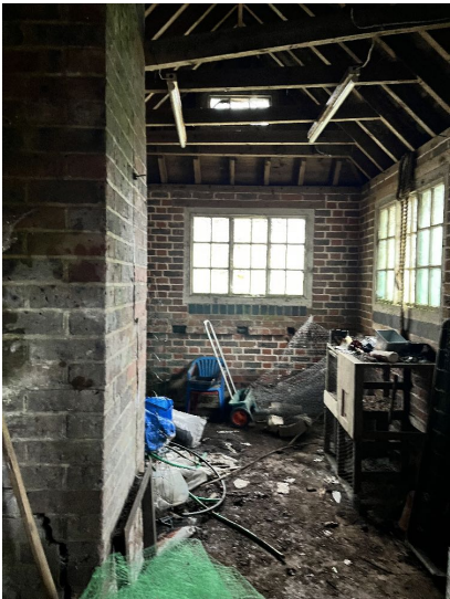
IM03 - Internal view looking north
