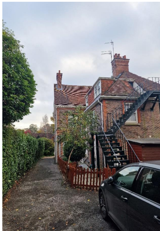
Rear (north) elevation showing shared driveway and external steps to flat 16c.
