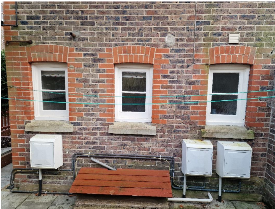
It is intended that a rear window (far right) is replaced by an external Victorian-style door.
