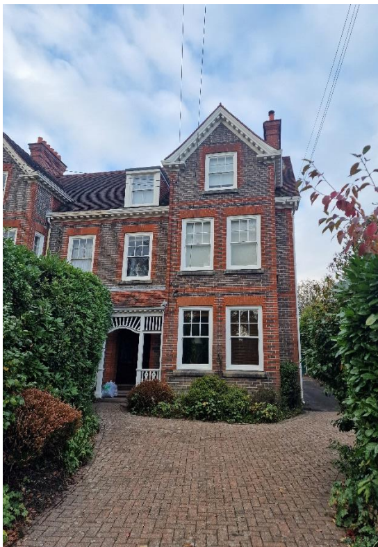
South (principal) elevation. Flat 16a is on the ground floor.
