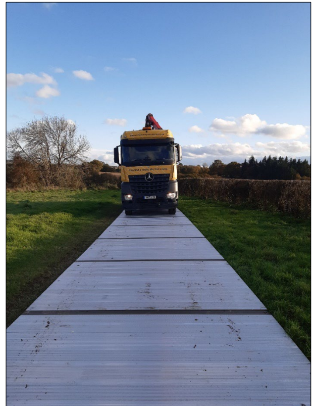
Figure 5 Example of Trackway System in use
