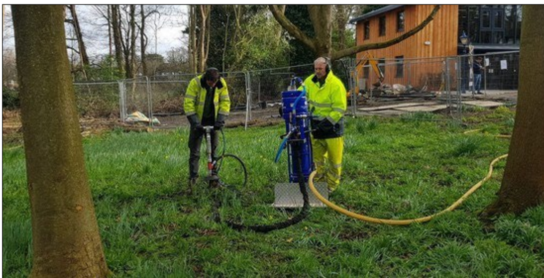
Figure 4 Air Injection Decompaction being carried out by a team from Ruskin
