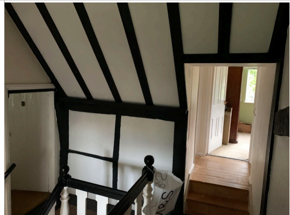
View of first floor stair landing
