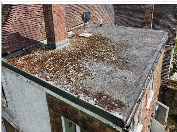
Flat roof to 1970 extension
