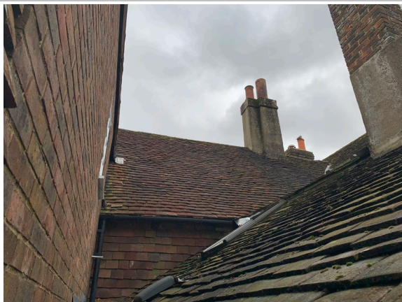
Rear roof slope and chimney stack of the original roof
