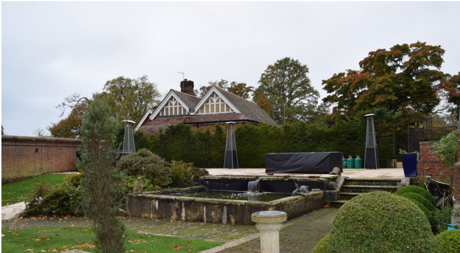
Figure 86 - The Site - Stonehurst Country House - reinstating conservatory
