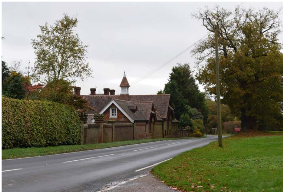
View looking southeast from the delivery entrance to Wakehurst Place (North Drive), adjacent to 1 & 2 Yew Cottages (Viewpoint 37)
