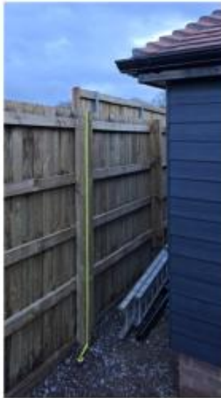
Photograph 1 Denton Homes 2.5m high acoustic fence
