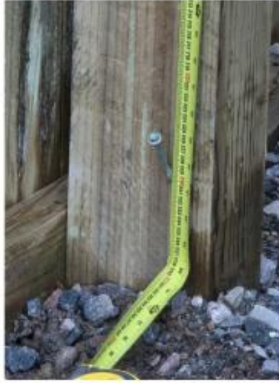
Photograph 2 Denton Homes 2.5m high acoustic fence
