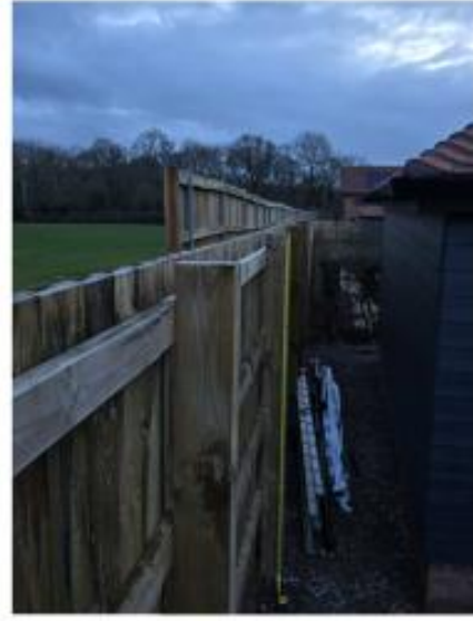
Photograph 3 Denton Homes 2.5m high acoustic fence
