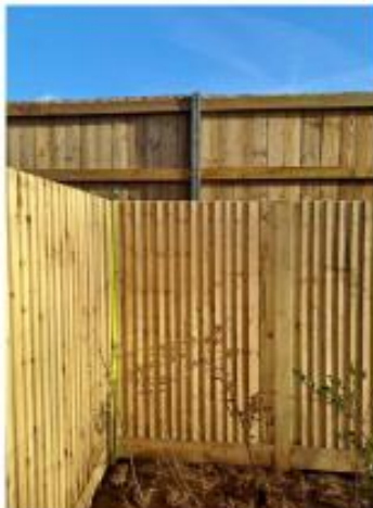
Photograph 5 Denton Homes 1.8m high fence
