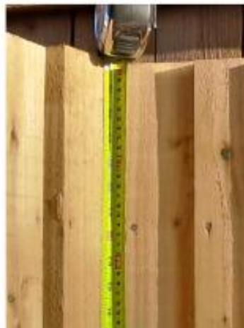
Photograph 6 Denton Homes 1.8m high fence
