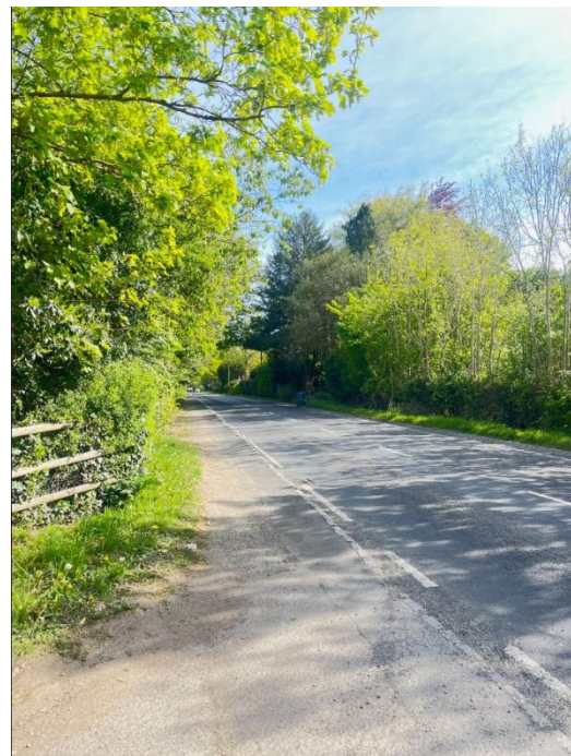
Figure 10 – South visibility splay onto Turners Hill Road
