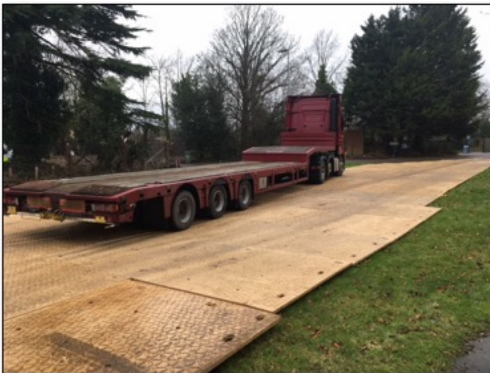
Fig.2 Heavy-duty metal ground plates laid on minimum 75mm depth sharp sand/ woodchip, fixed in position with road pins.
