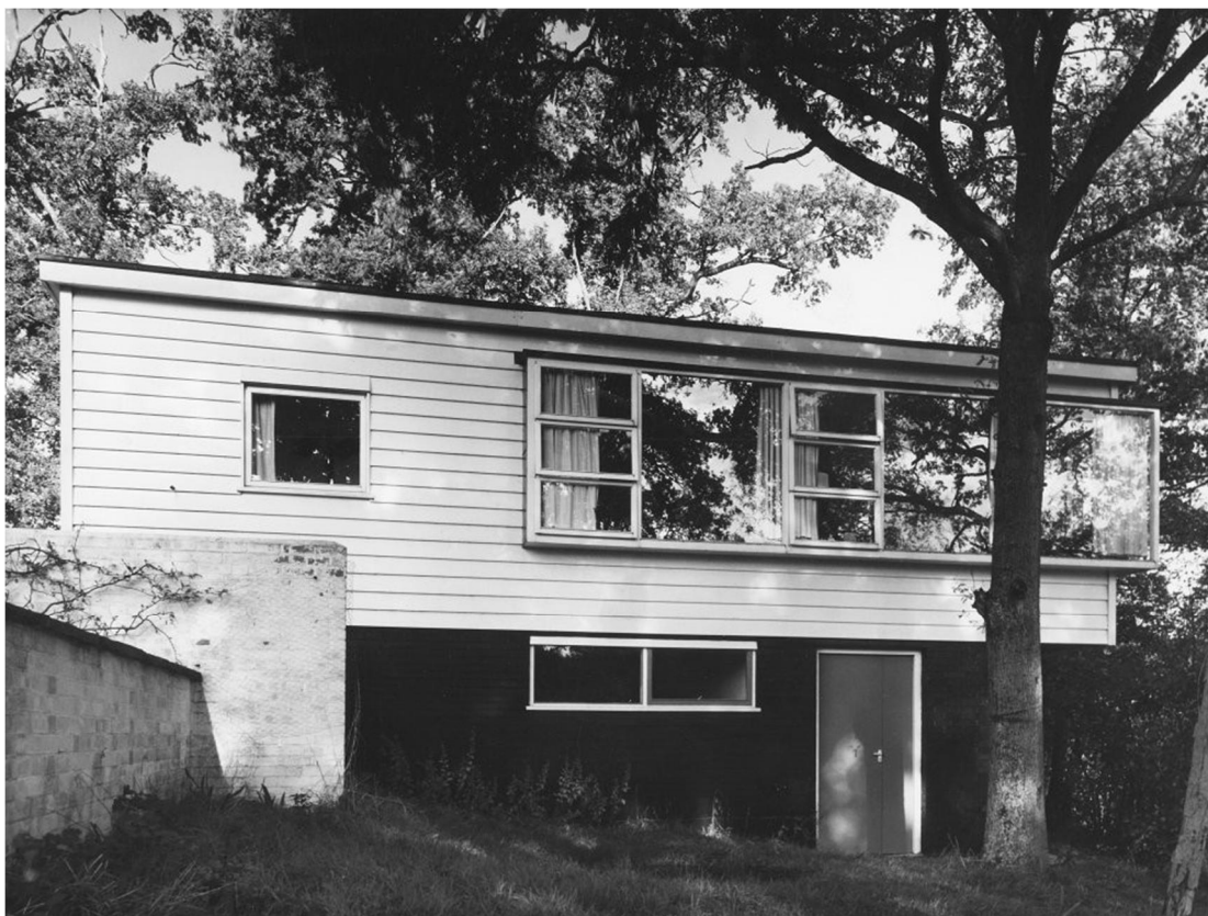
Photos taken when Annexe was new (1960's) showing the slope down to The Mill Pond
