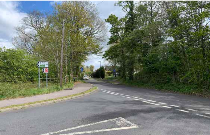
Hurstwood Lane access from relief road Photo 8
