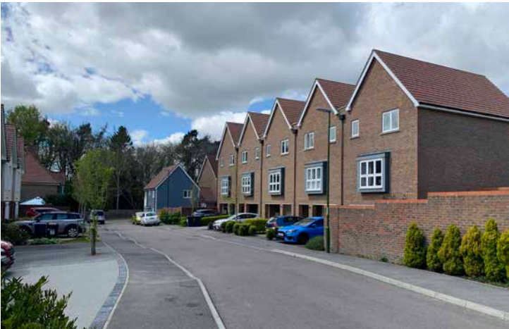
Woodside 3 storey townhouses
