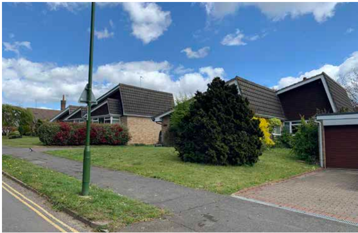
Asymmetrical Roofs (Hurstwood Lane Greenhill) Photo 1
