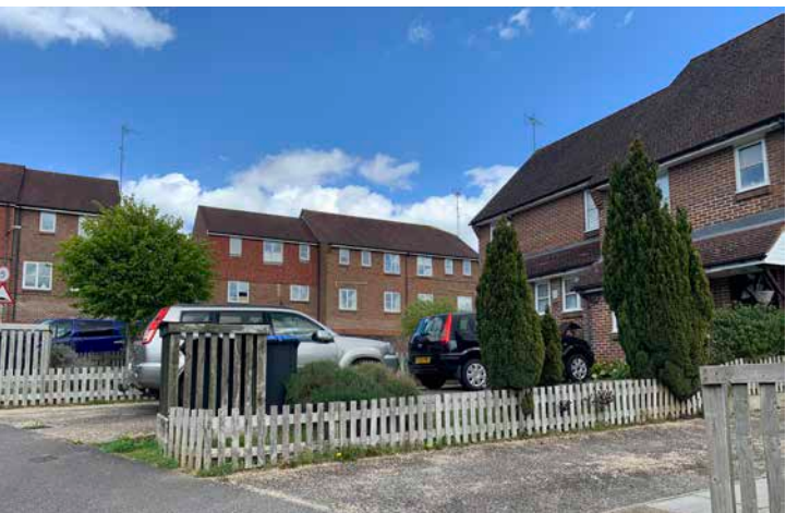
Woodside houses with integrated garages
