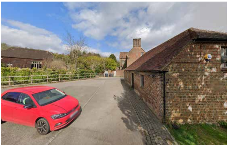
Existing building in Hurst Grange Photo 5
