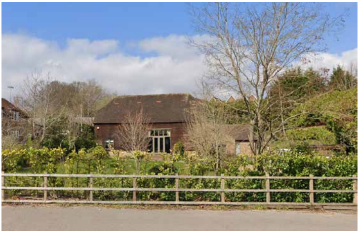
Hurst Barn Photo 6
