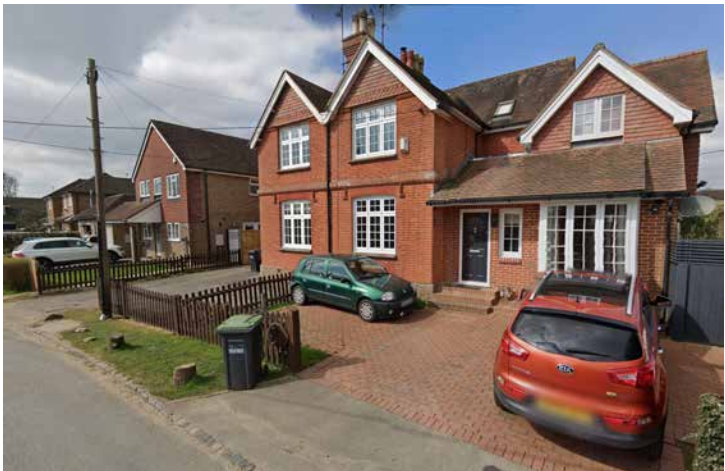
Woodside houses with integrated garages
