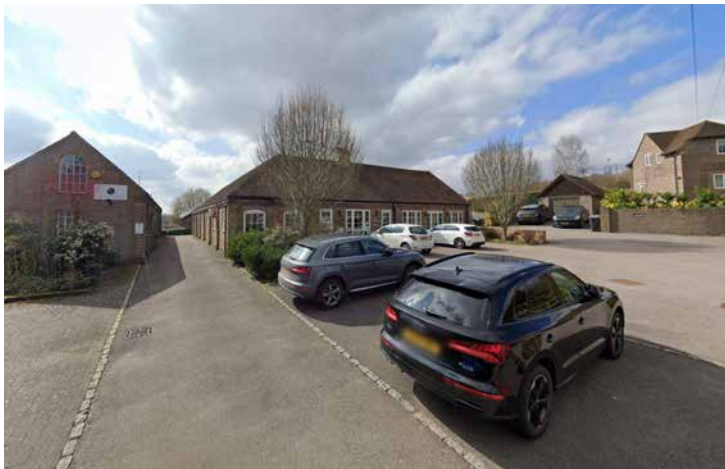
Hurst Grange business units and cottages Photo 3
