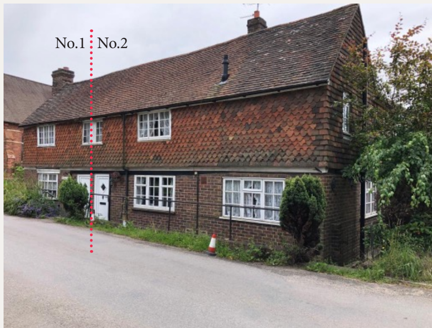
Figure 3: Brickyard Cottages viewed from the west, showing the additional bay at the west end added in the late 1970s
