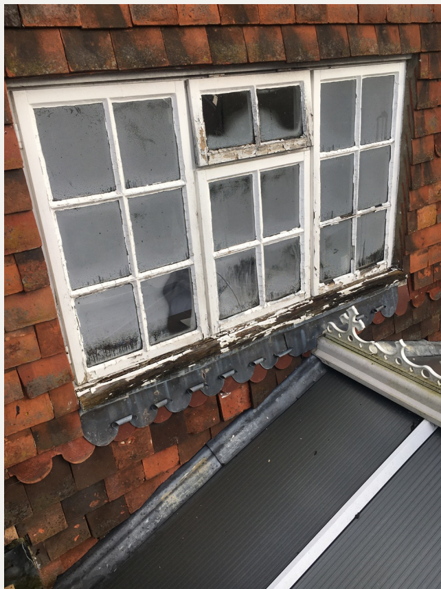
Figure 8: Typical existing storm-proof casement – in this case window 11
