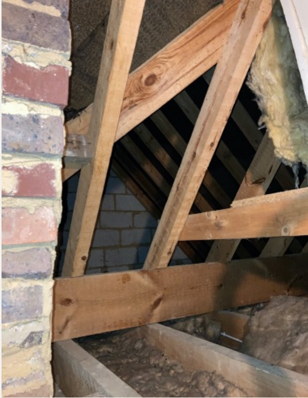
Figure 5: modern roof timbers and ceiling joists, brickwork and blockwork. Chimney stack at extreme left, looking towards the garden-facing gable over Bedroom 2
