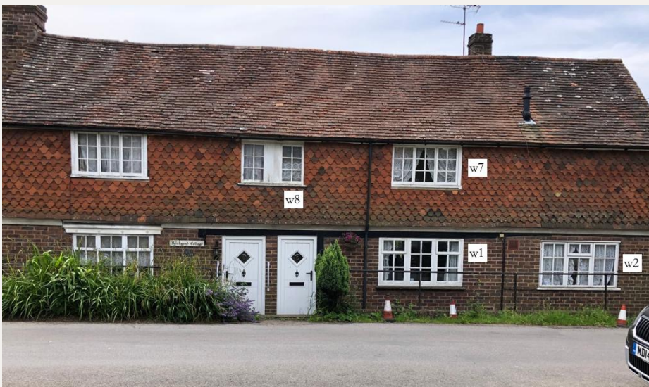
Figure 6: Elevation to Street Lane illustrating glazing types. No2. Brickyard Cottages is in the right-hand part of the building. The window to the left of No1's front door is a shallow bay.
