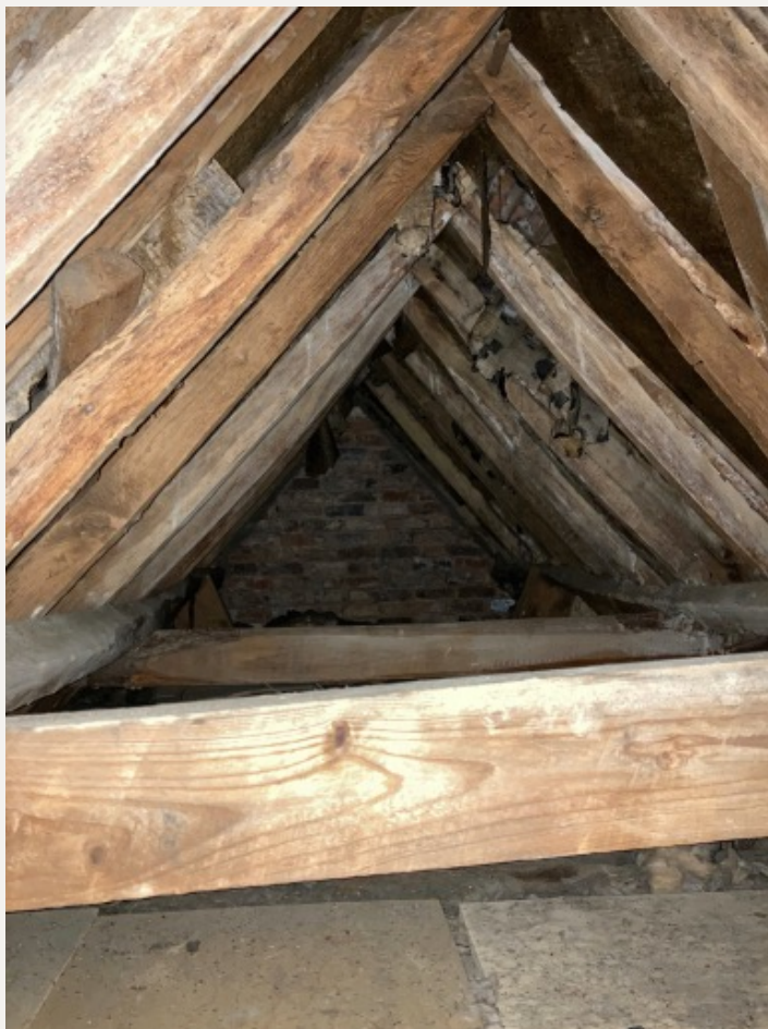
Figure 4: Looking towards the party wall with No.1 Brickyard Cottages from a position roughly in line with the chimney stack in No.2, showing a mix of old and new timbers in the roof.
