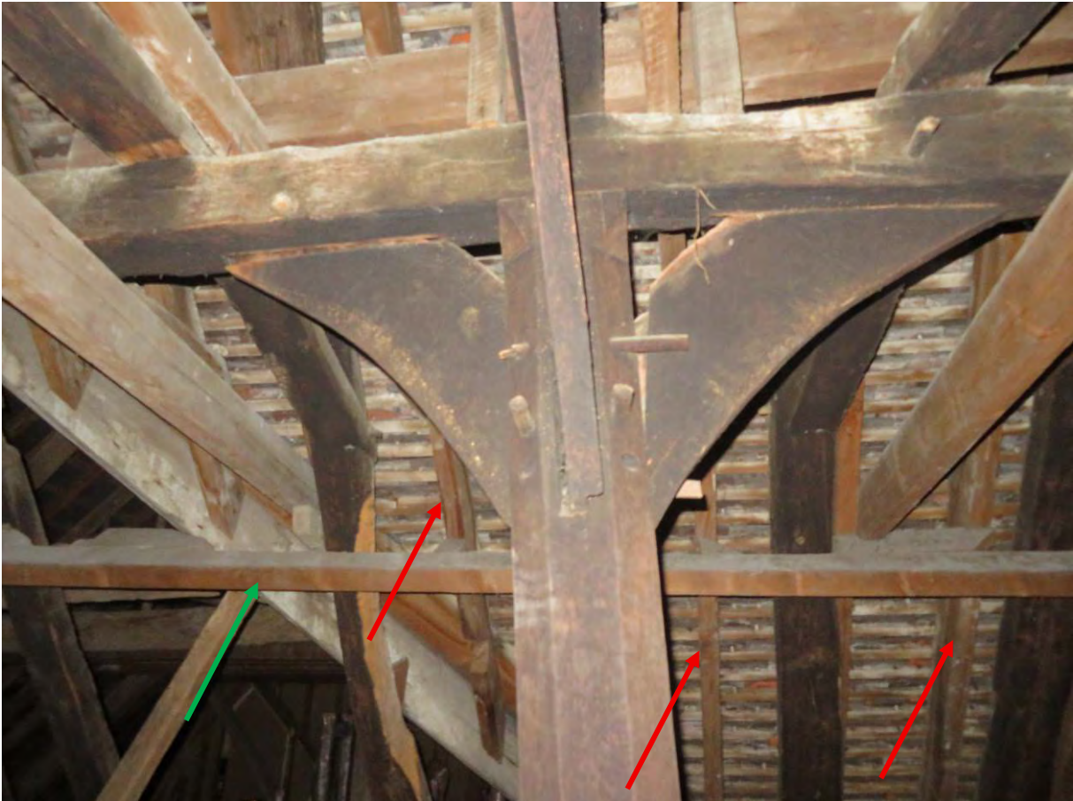
Photograph 8: Modern rafters to east of Bay 2/3 (red) and purlin (green)
