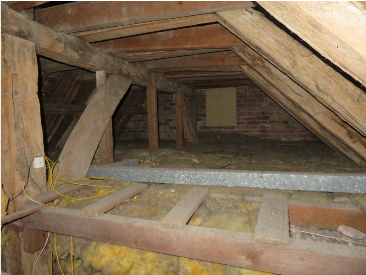
Photograph 15: Bay 1 roof structure
