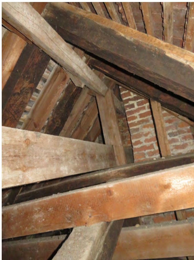
Photograph 9: Added frame above collars purlins to Bay 3 and 4
