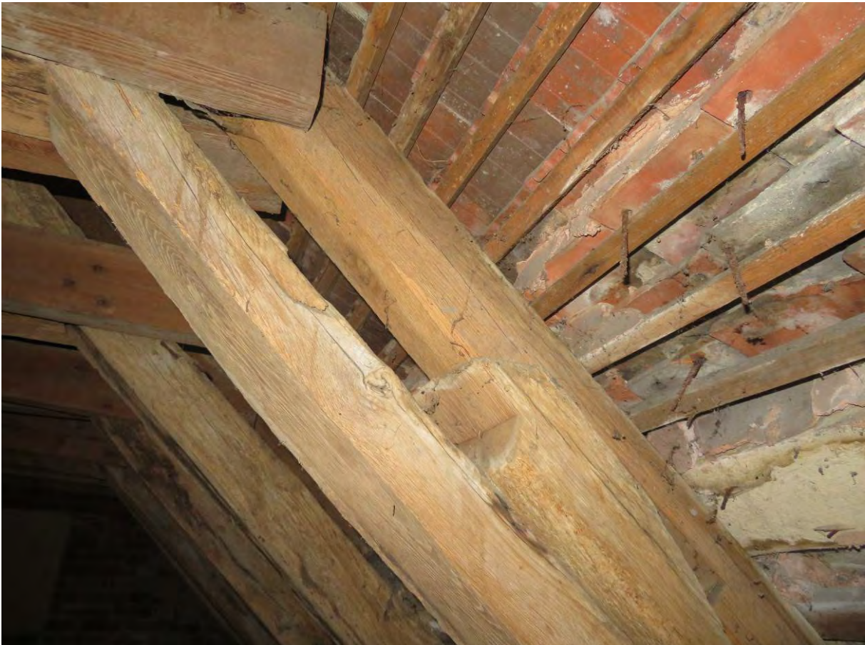
Photograph 16: Outer rafters to west elevation to Bay 1 and 2
