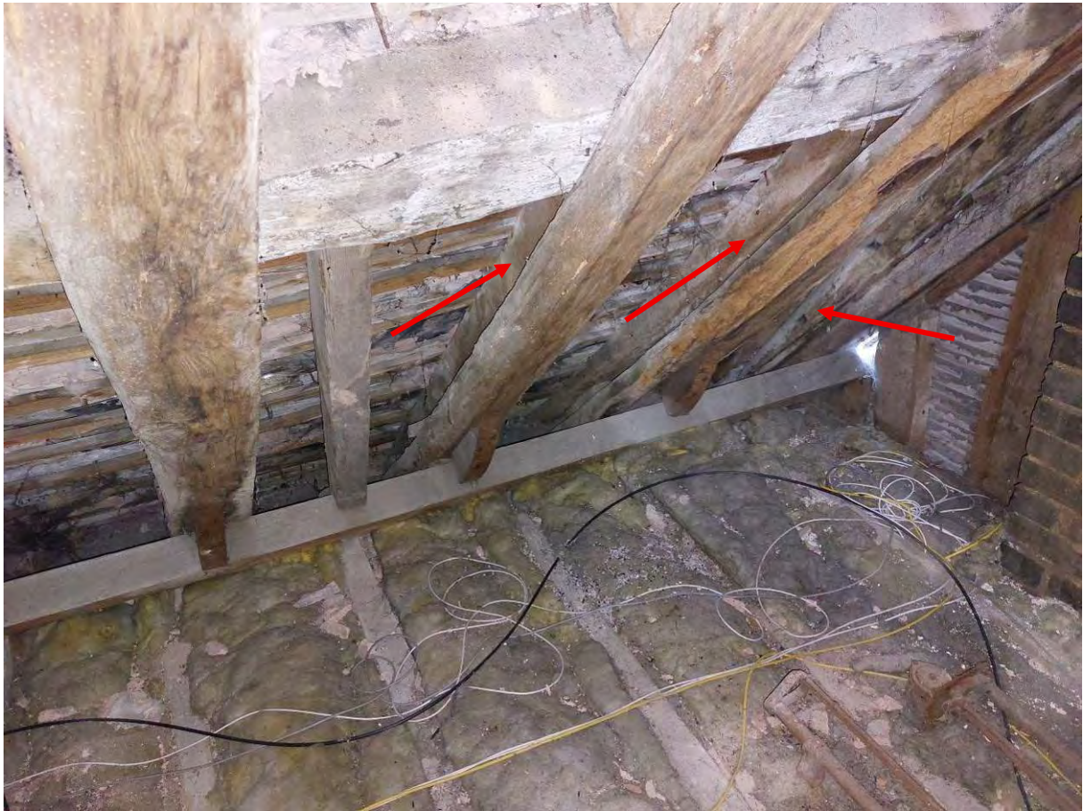
Photograph 5: West elevation of Bay 5 with added rafters over originals
