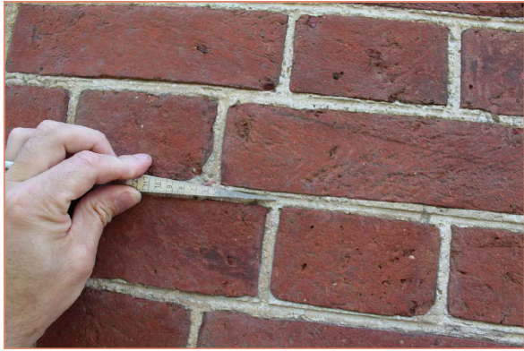
The front elevation displays limewashed areas and also "penny rolled" pointing
